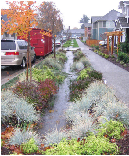
Bioswales help reduce stormwater runoff
