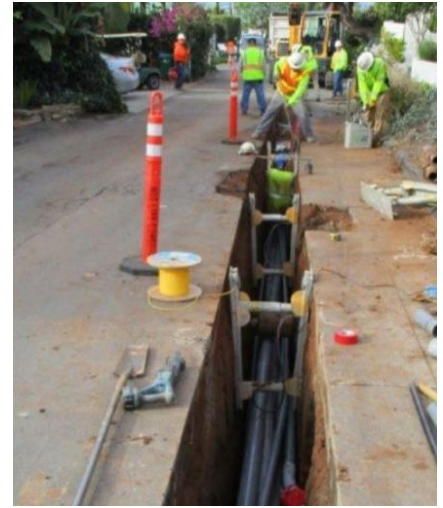
Work to underground utility poles and wires
