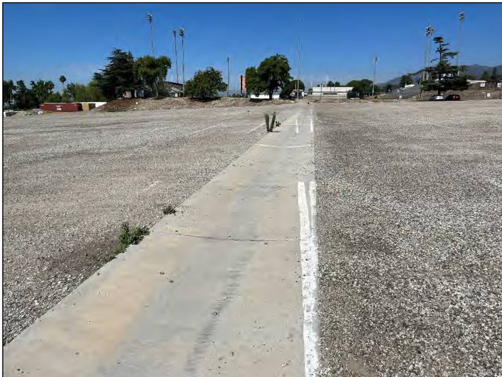
Looking south at the concrete lined ditch of Drainage A.
