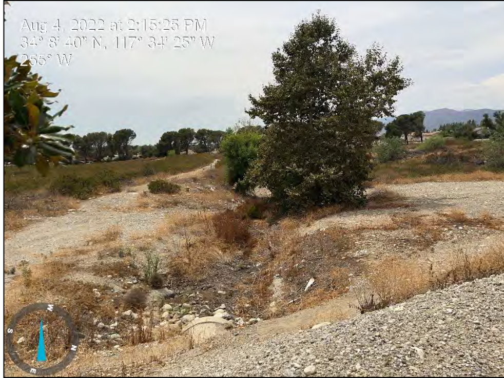
Downstream portion of Drainage B prior to the detention basin.
