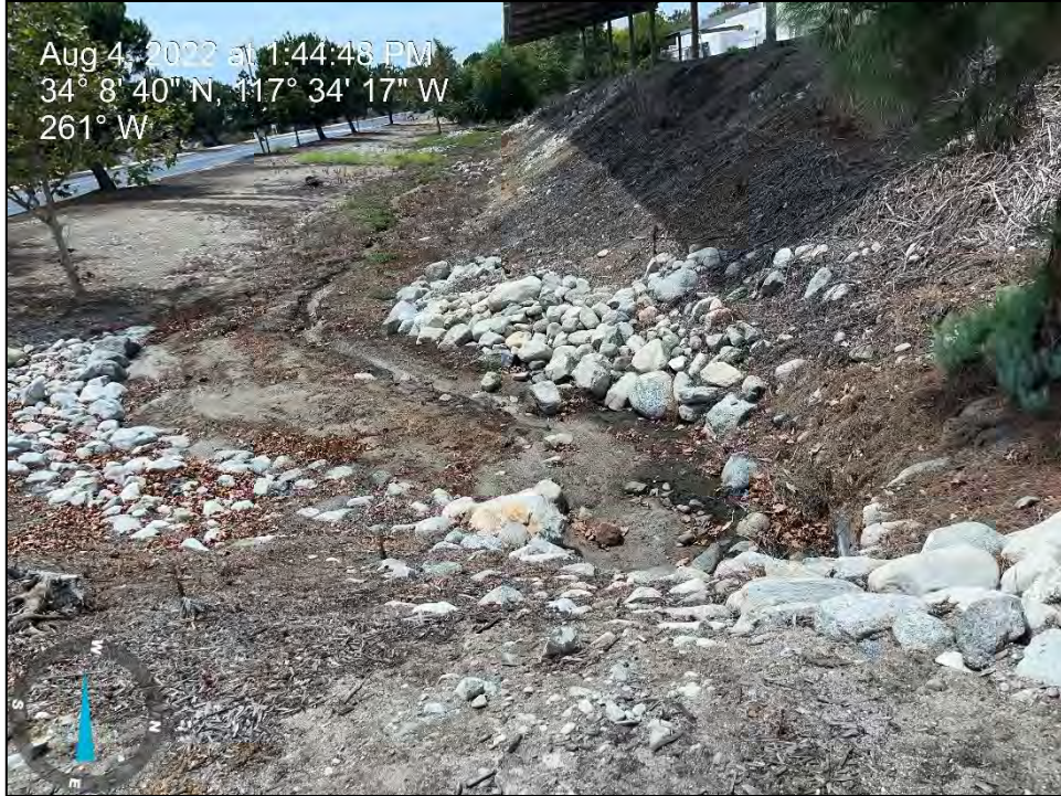
Looking west at the downstream portion of Drainage B.
