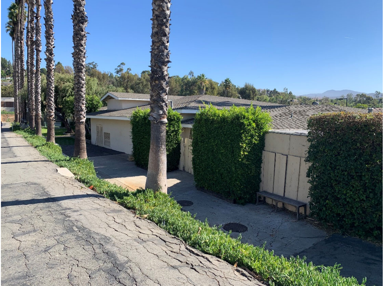
Clubhouse, northwest elevation, facing south
