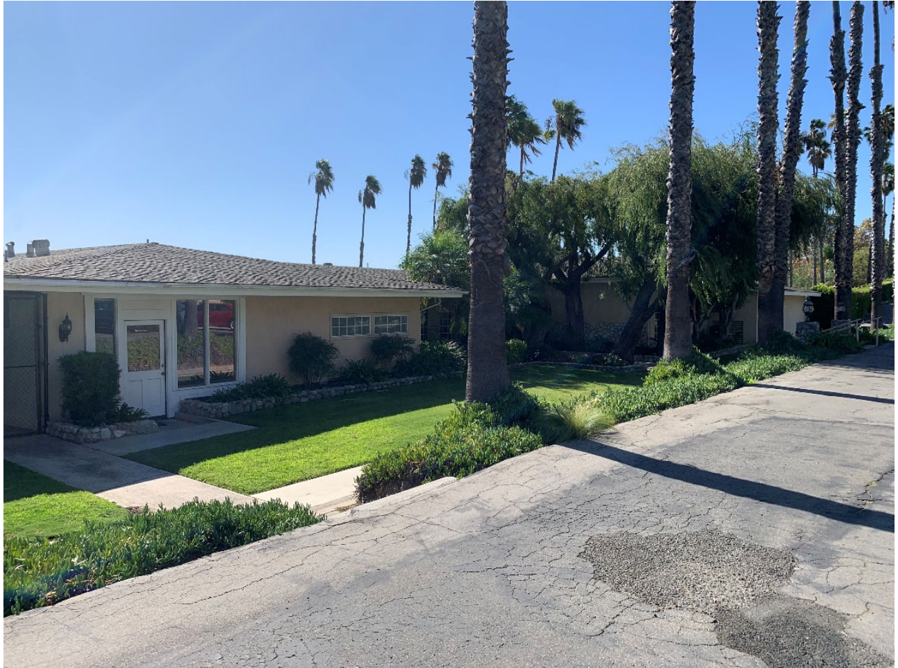
Clubhouse, northwest elevation, facing south
