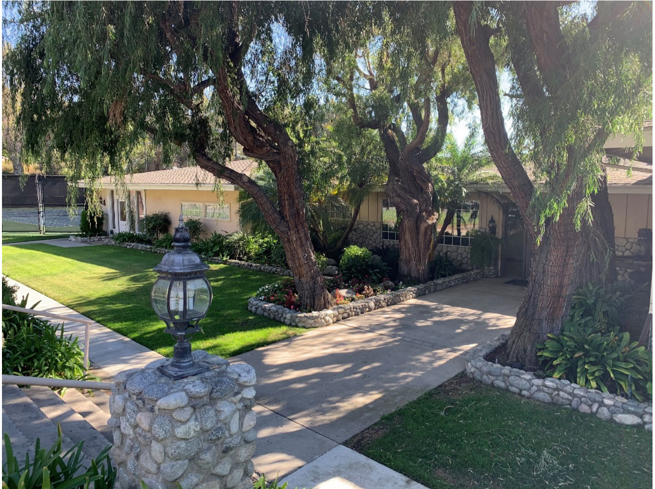
Clubhouse, northwest elevation, facing north
