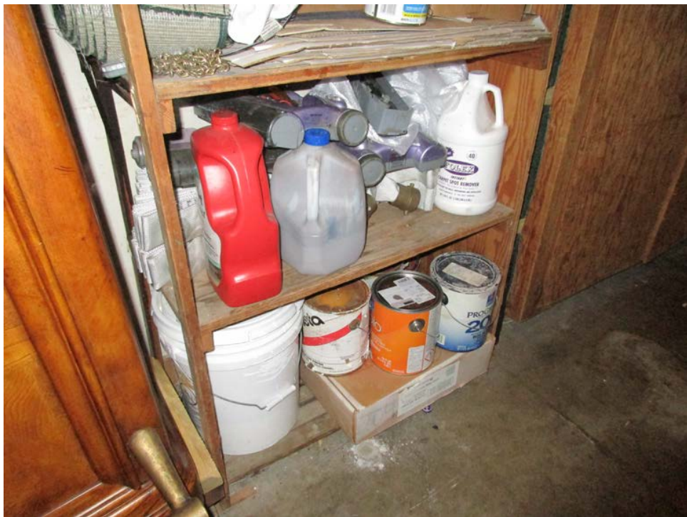
Photo 8 – Paints and cleaners storage in the hot water heater room in the clubhouse.
