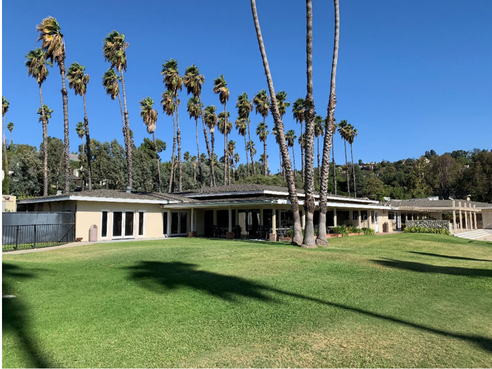
Figure 5-1 Clubhouse, southeast elevation, facing north
