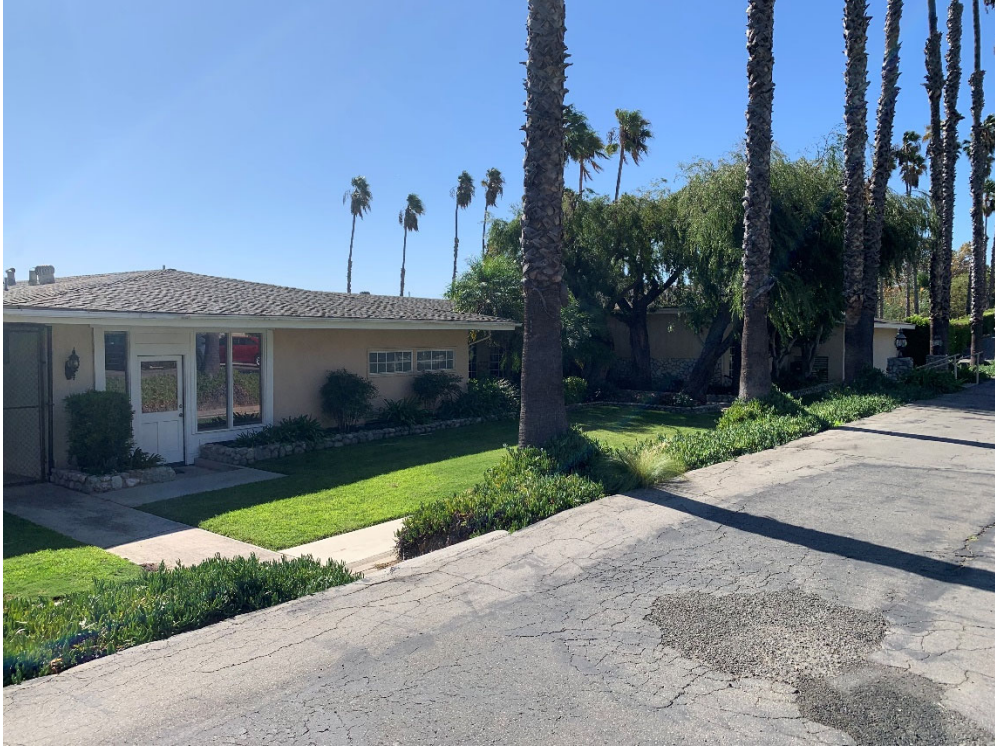
Figure 5-3 Clubhouse, northwest elevation, facing south
