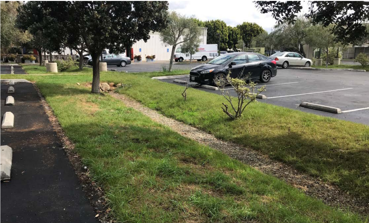
Photograph 2. View of a bioswale in a developed area of the biological study area. Photograph taken near the southeastern boundary of the project site facing northeast.
