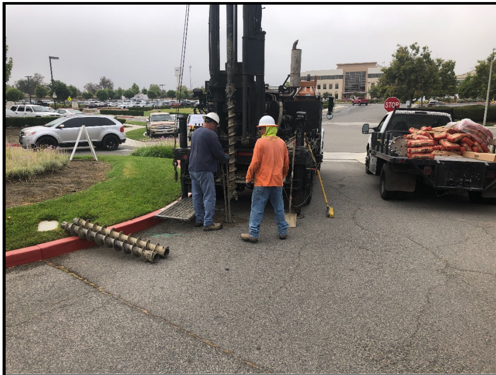
Figure 3-2. Drilling Geotechnical Test Boring B-1
