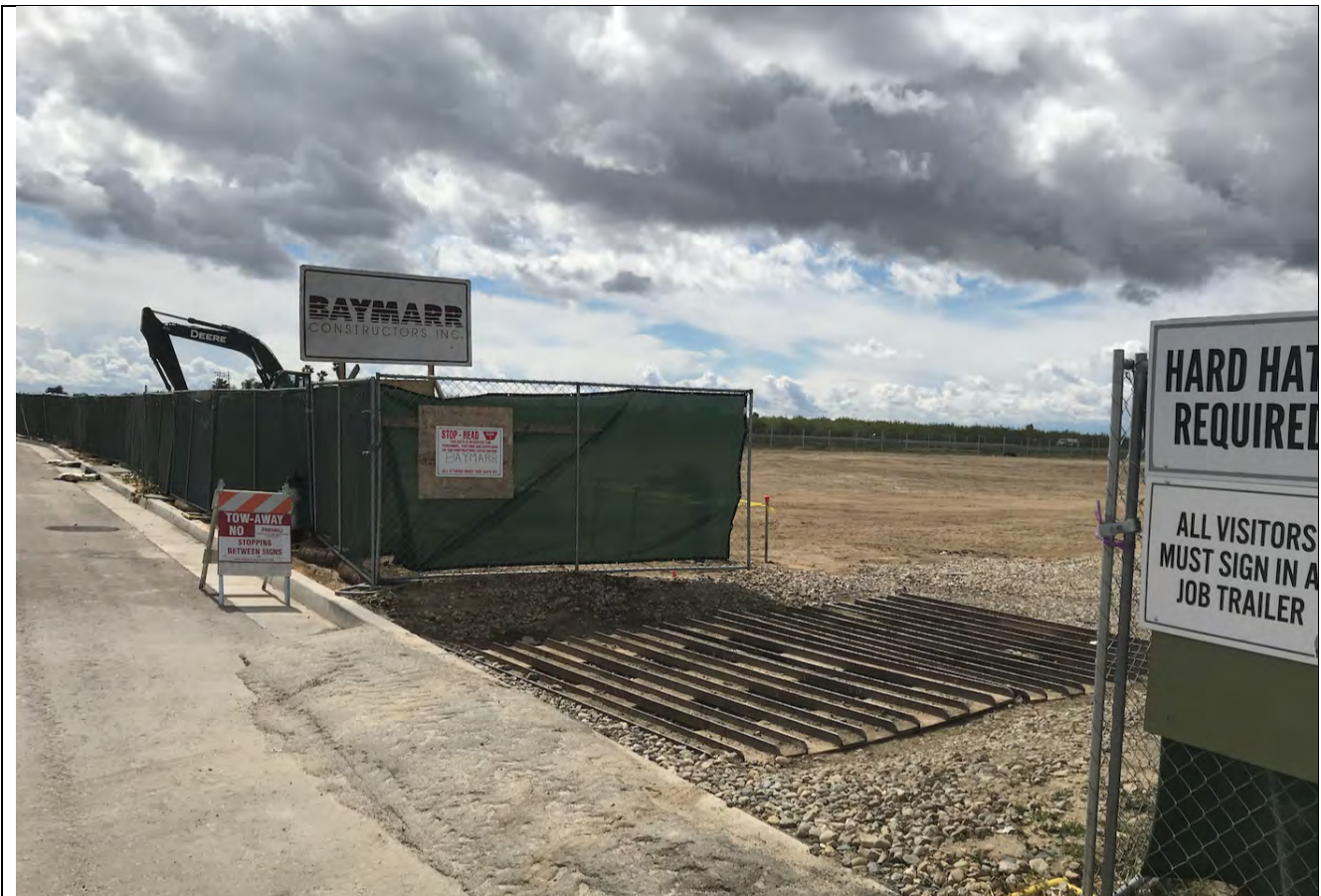
Photo 1: View south from Northpoint Avenue toward Study Area and construction entrance.
