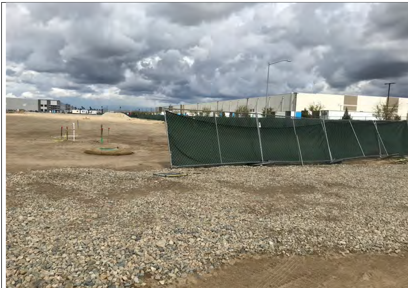
Photo 5: View of northern edge of Study Area. Gravel area is part of construction entrance.
