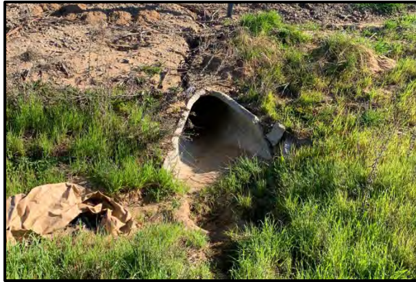
Photo 3. Stormwater culvert between Study Area and Highway 101 southbound, view east. January 20, 2022.
