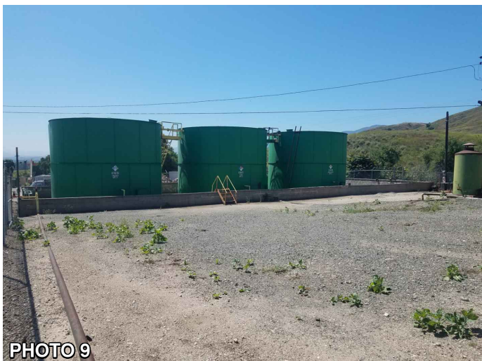
AST AREA - STOCK TANK, WASH TANK, AND DISPOSAL TANK
