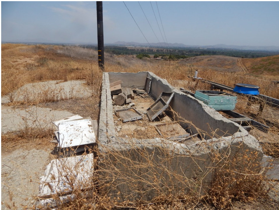
Plate 3. Concrete slab and debris-filled trough at SH-S-002. View to the west.
