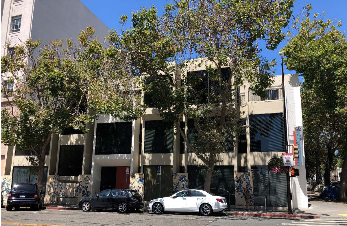
Figure 5 2118 Milvia Way, South Elevation, Facing North
