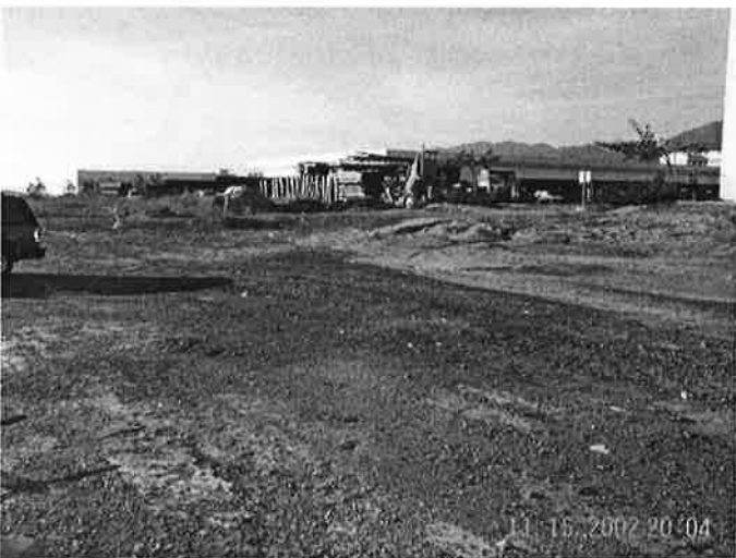
5. Slag-gravel graded parking area in the northeast quarter of the site (view northwest).
