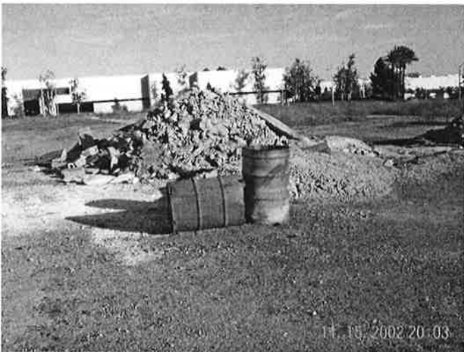
3. Concrete waste and construction debris, two drums filled with rags and trash in northeast quarter of property (view east).
