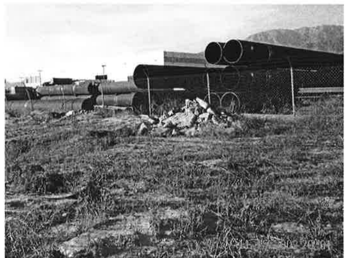
4. Concrete rubble on the north edge of the property next to the steel pipe storage area on the adjacent site north (view north).
