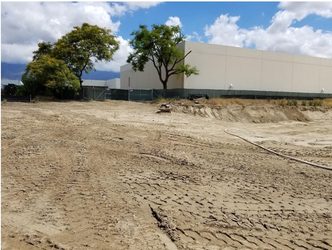
June 29, 2020 - Looking North, excavation complete (storm drain manhole exposed above grade)
