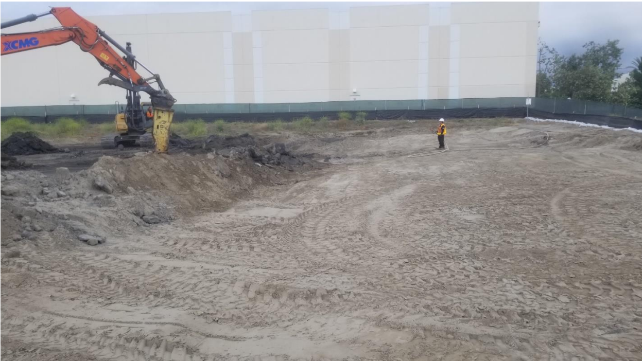
May 18, 2020 - looking North as excavation progresses westward
