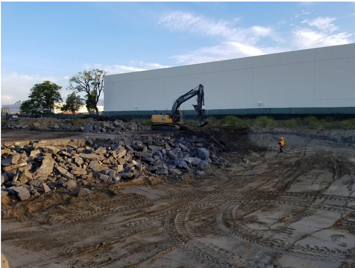
June 1, 2020 – looking Northwest at excavation progress
