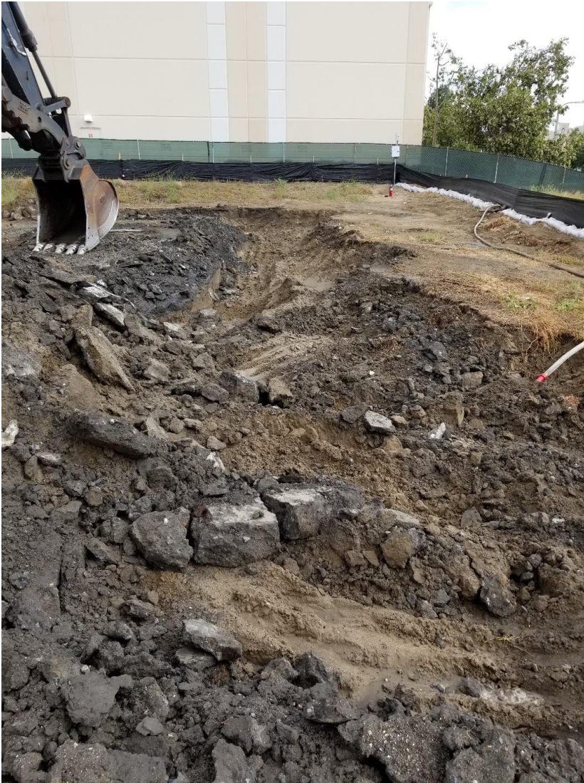
May 11, 2020 looking North along eastern edge of excavation
