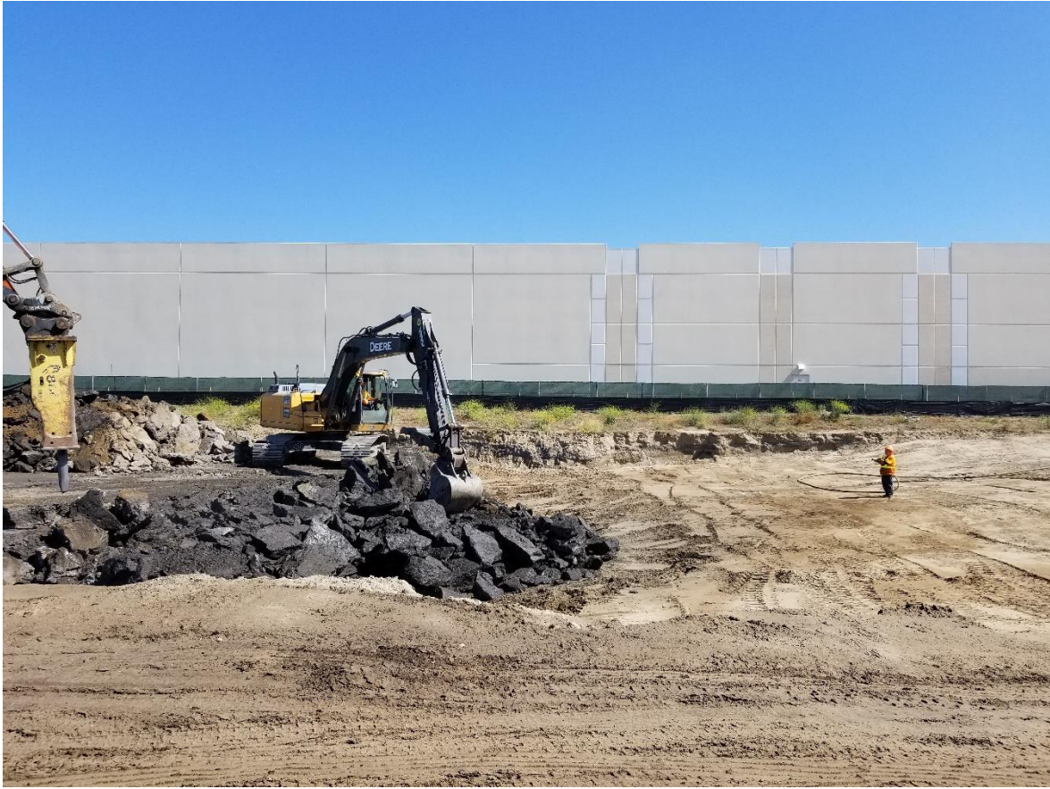
May 26, 2020 – looking North at excavation progress
