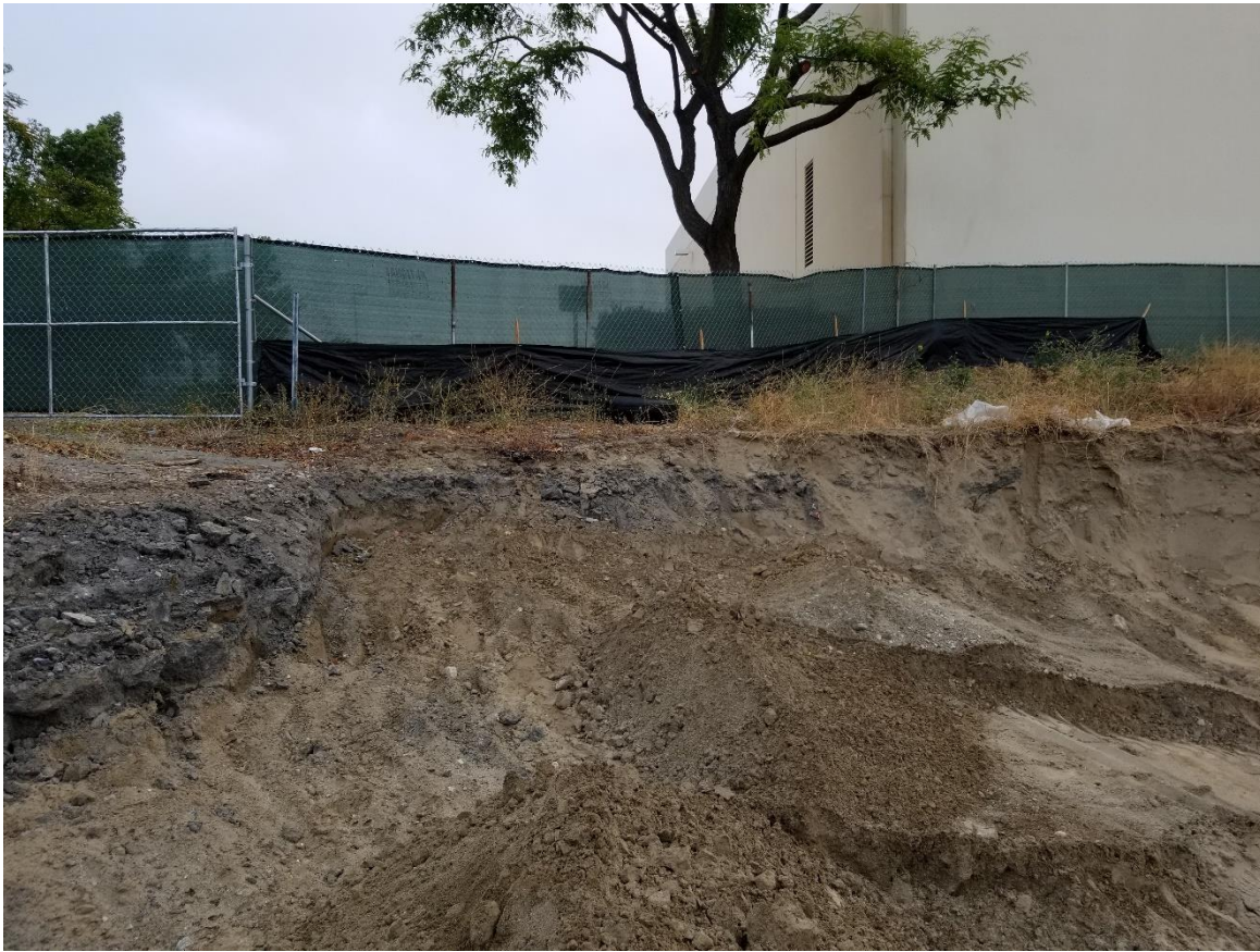
June 22, 2020 - looking North at excavation progress
