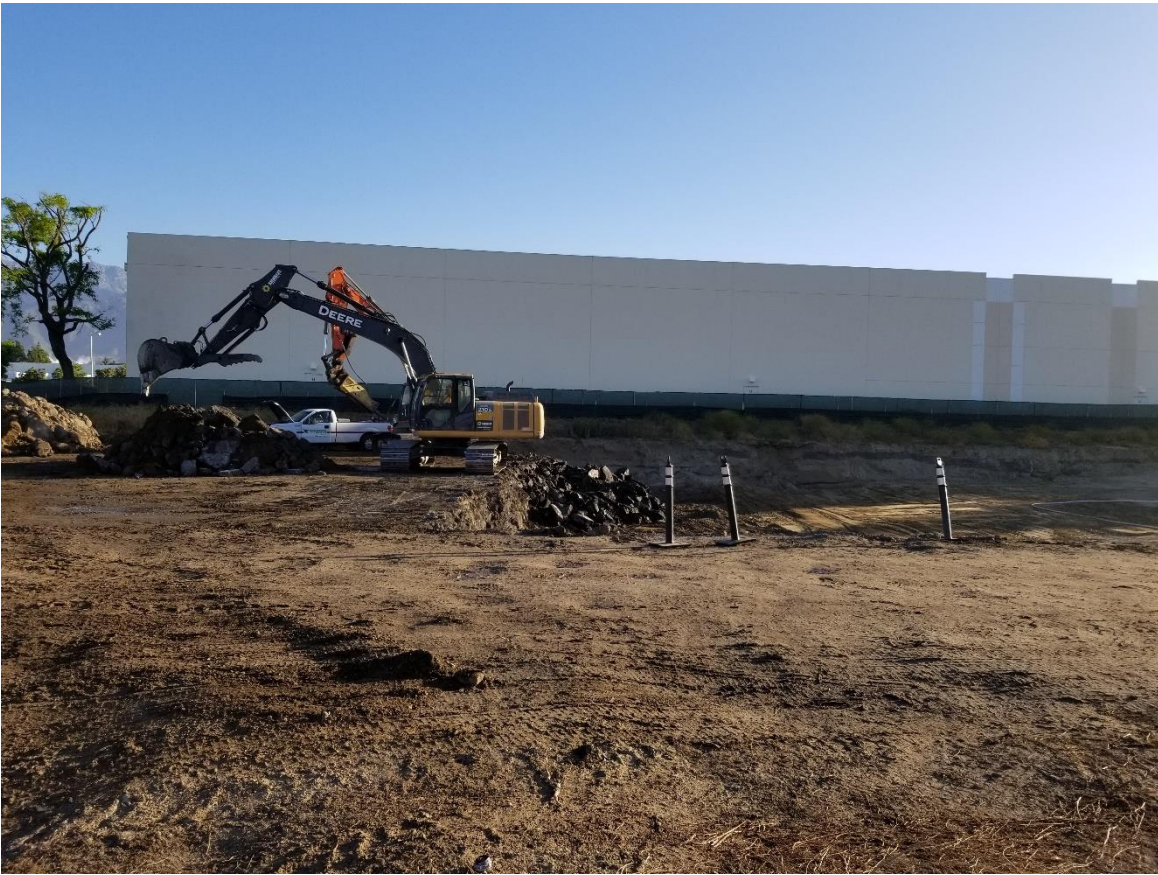
June 8, 2020 - looking North at excavation progress
