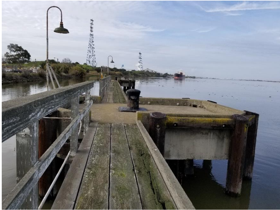
Figure 5. West end walkway and mooring docks, facing west-southwest.
