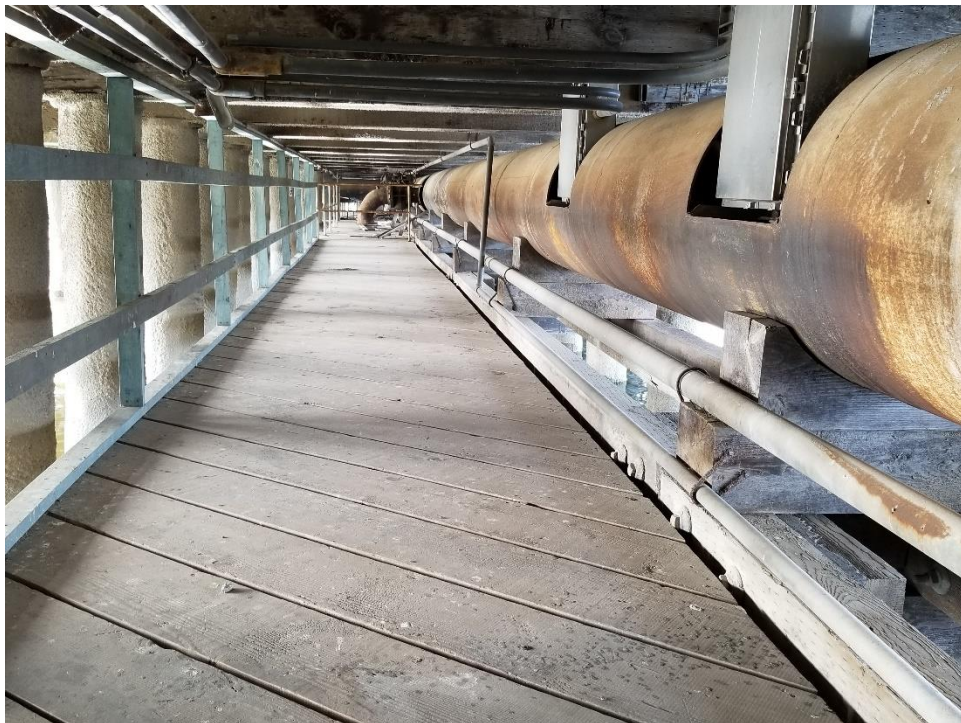
Figure 10. Walkway and pipeline below concrete deck.
