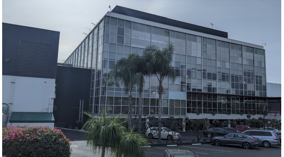
Image 2: North Facade of Service Building
