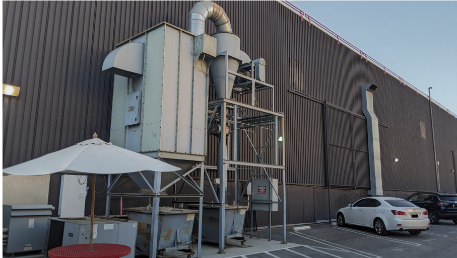
Image 5: East Addition Facade and Equipment
