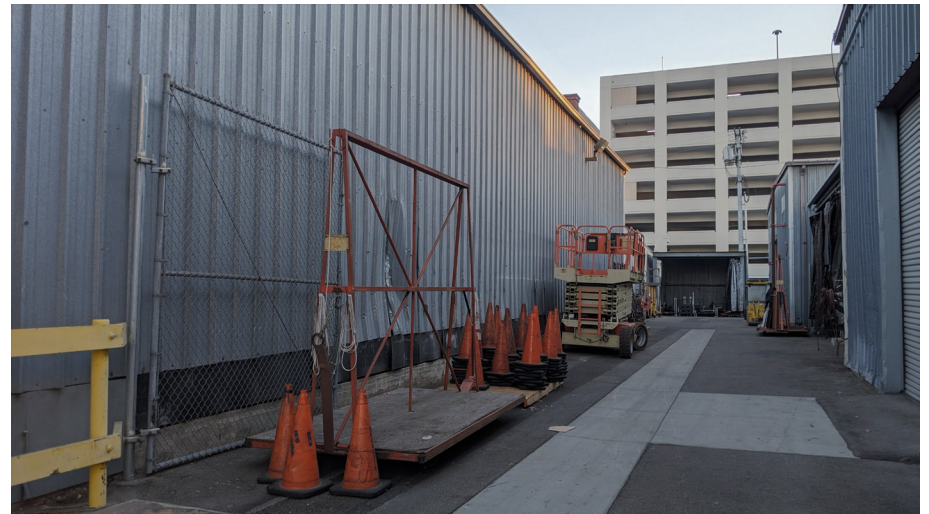
Image 8: Southeastern Site Corner with Storage Sheds
