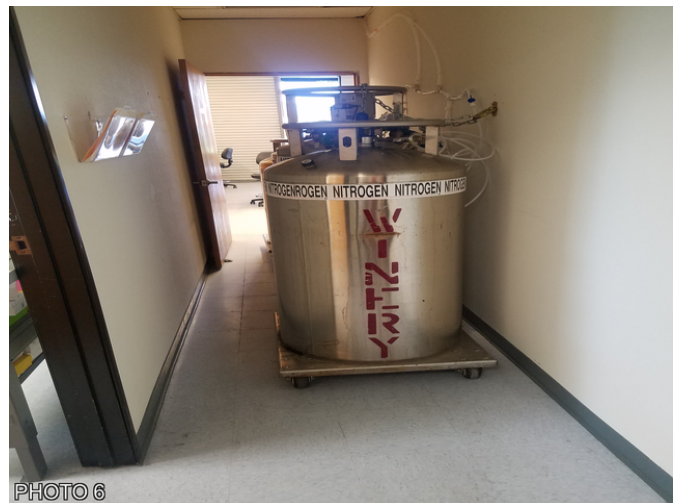
PHOTO 6 NITROGEN TANK IN 130G PRODUCE AVE
