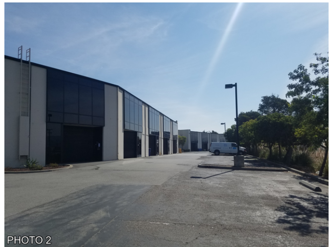
PHOTO 2 VIEW EAST ALONG SOUTHERN BOUNDARY OF PRODUCE AVENUE PARCEL
