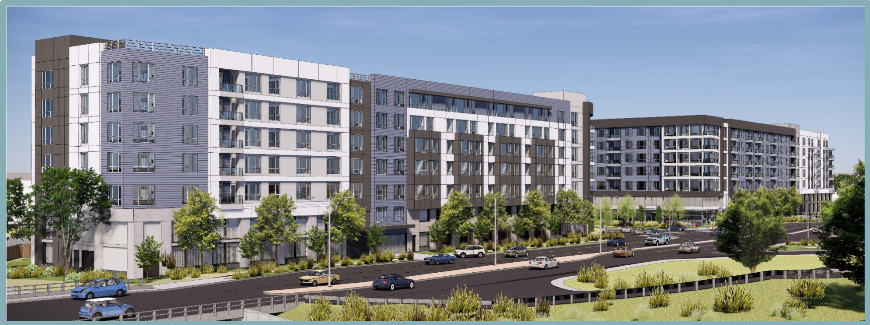
Figure 5 Completed Project, Looking North
