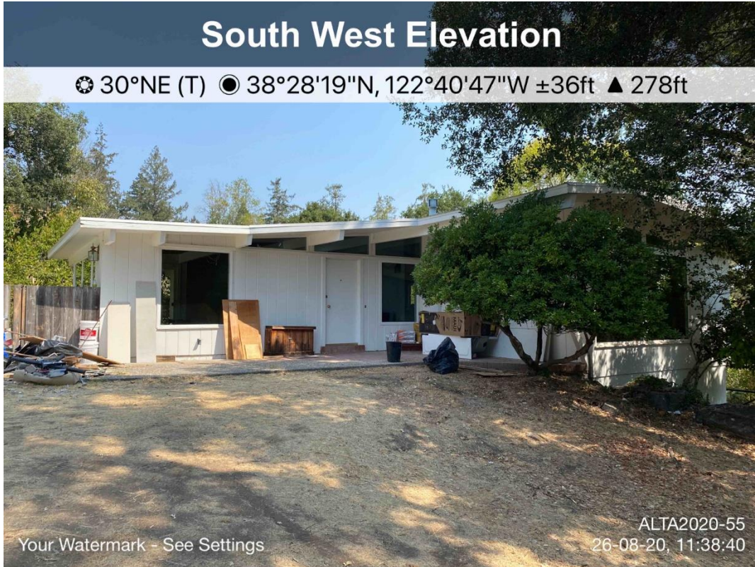
Photo 1: Front Elevation of Single-Family Home on Parcel
