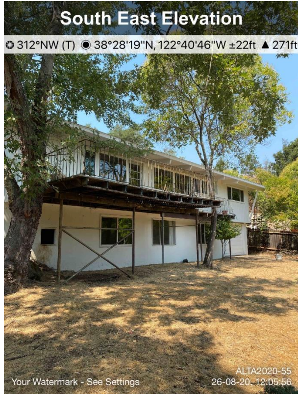
Photo 3: View of Single-Family Home from backyard
