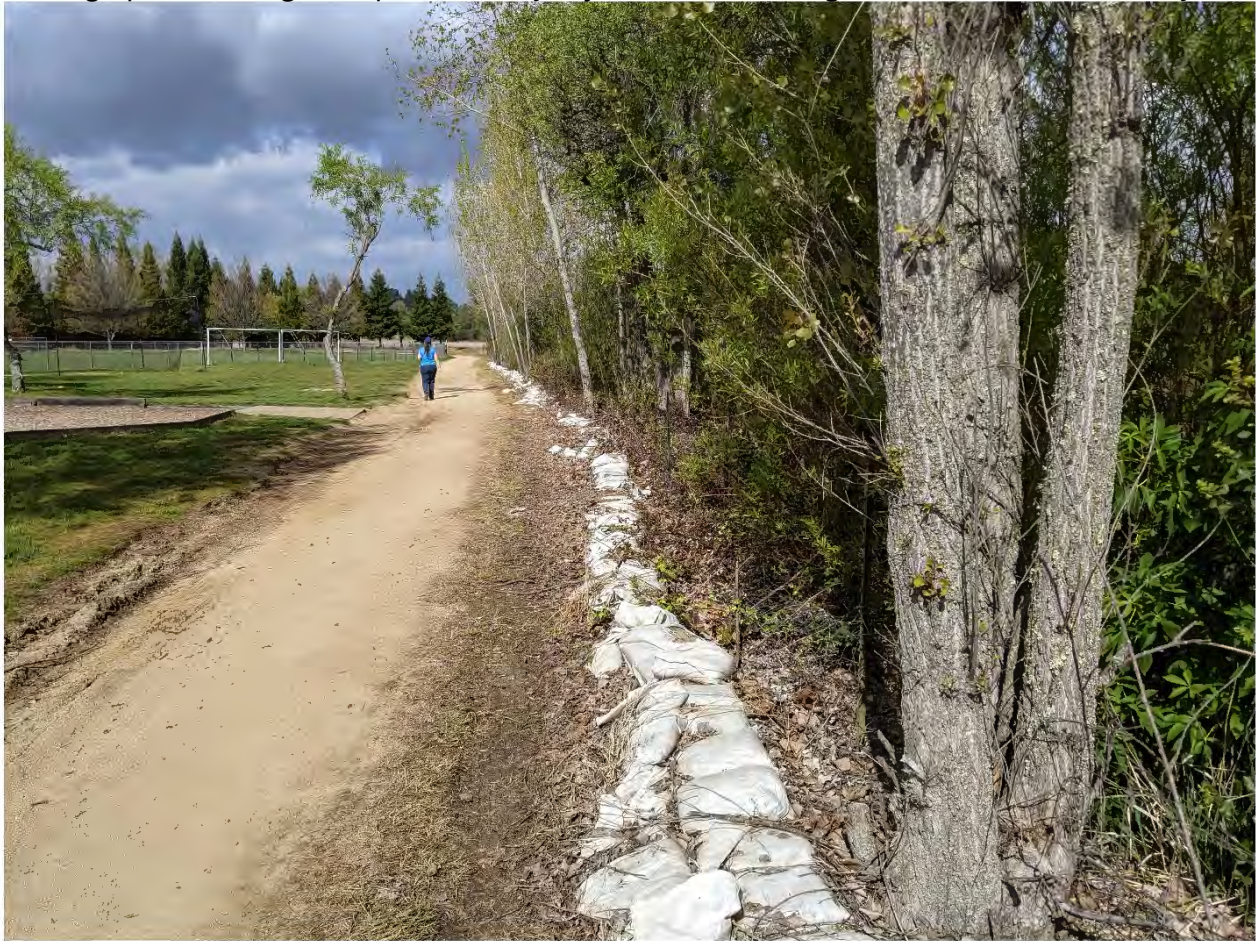
Photograph 2. Existing flood protection by adjacent stream along the southeastern boundary
