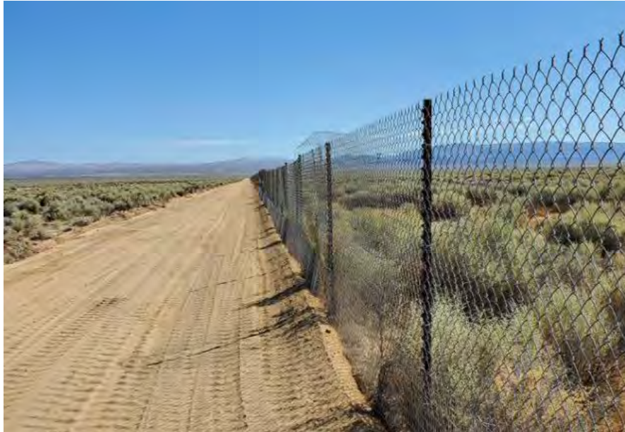
Boundary fence looking west
