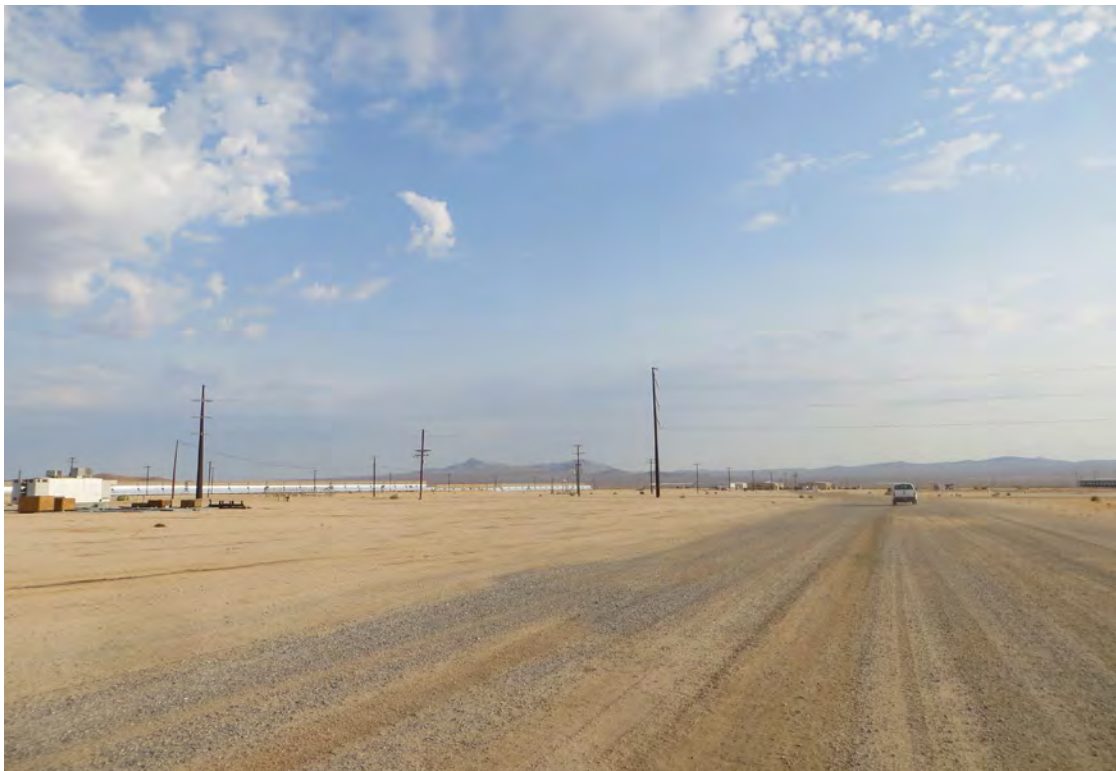
View of the Shared Facilities Area looking north from existing on-site access road.
