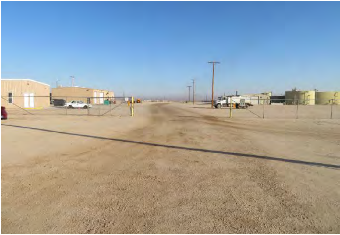
View looking north toward the southern portion of the Shared Facilities near Hoffman Road
