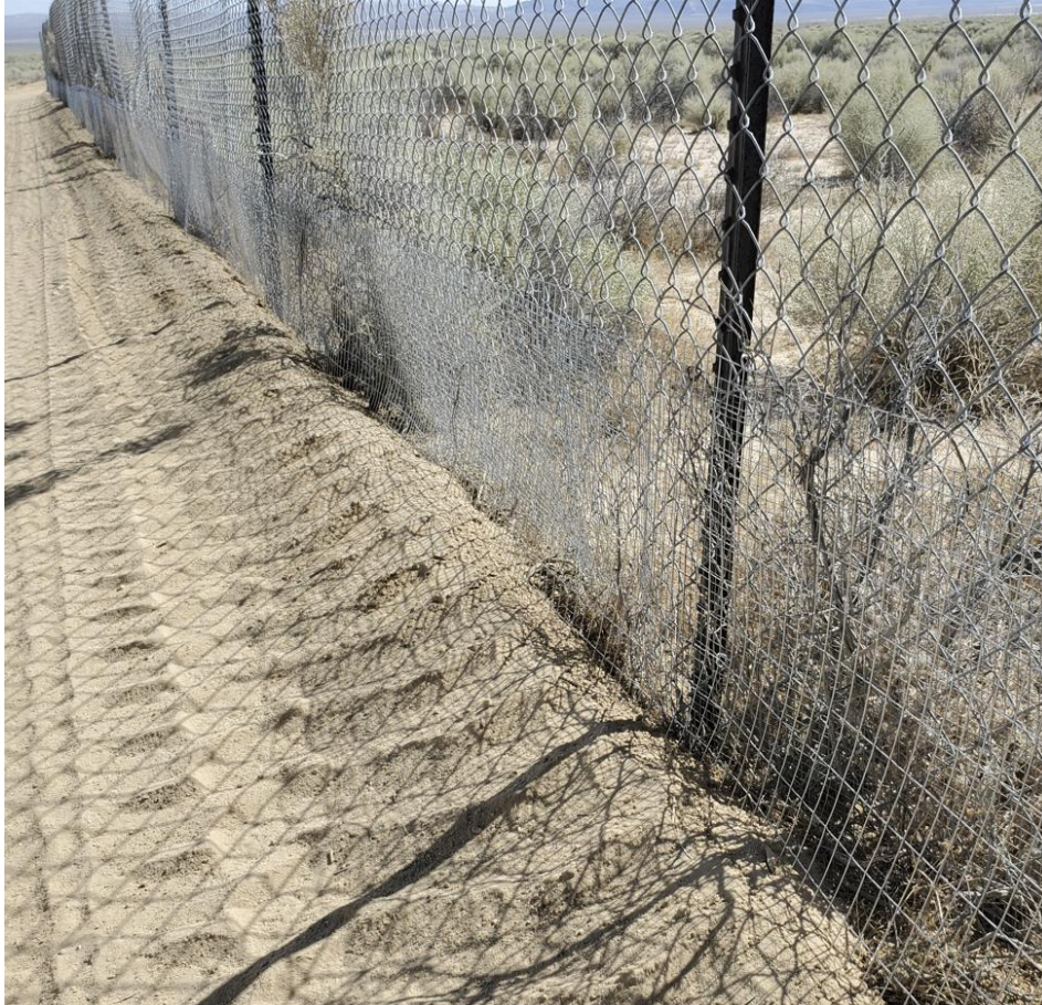
Photograph 23 – Showing the reinforced fence line with exclusion fencing.
