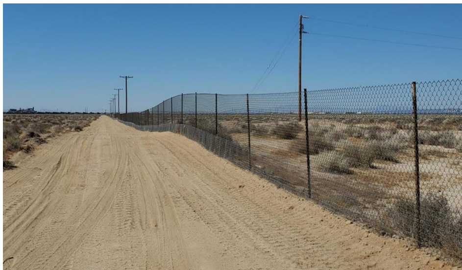
Photograph 19 – Facing south from the northeastern corner of the survey area at the reinforced fence.
