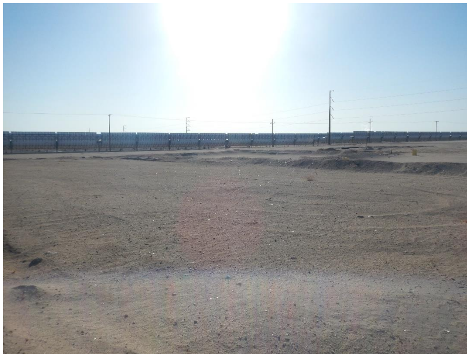
Photograph 21 – Facing southeast from within the Shared Facilities Area. This photo was taken in 2018 for the Lockhart Solar I Facility.
