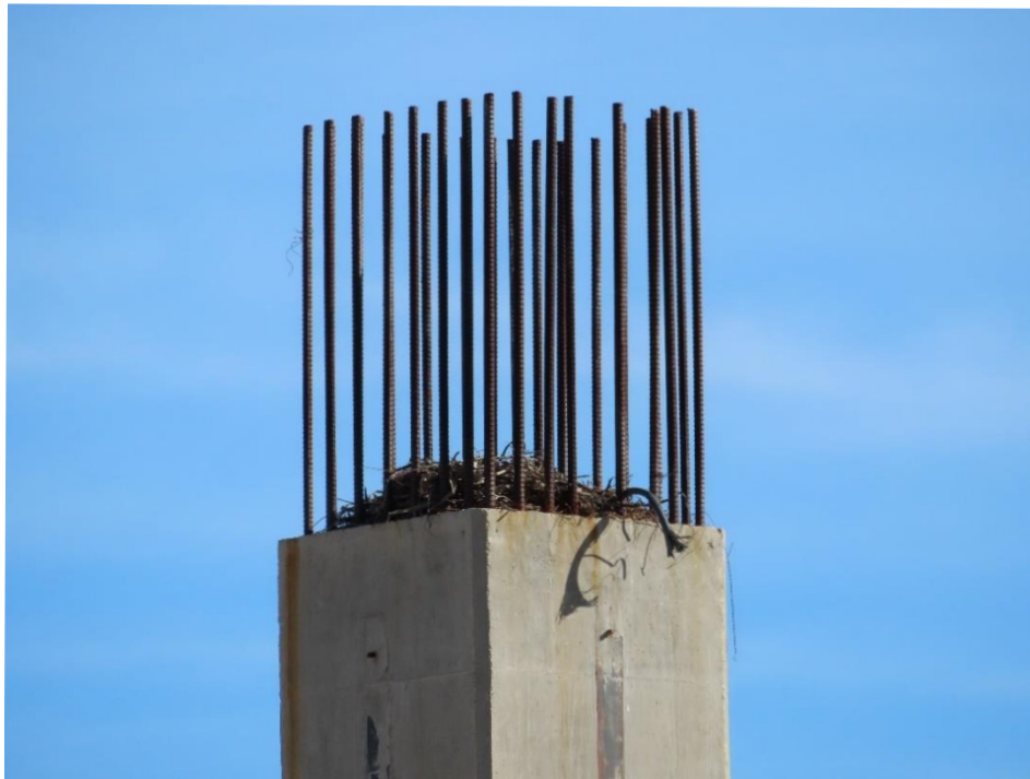
Photograph 2 – View of the remnant stick nest located within the concrete structure within the center of the survey area, facing northeast.
