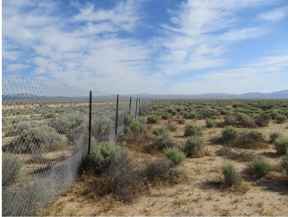
Photograph 7 – The majority of the project site is protected by both a chain link fence and desert tortoise exclusion fencing.
