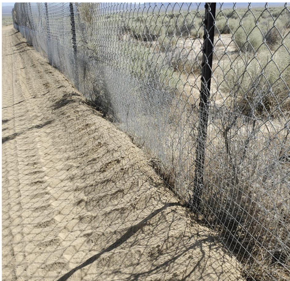
Photograph 20 – Showing the reinforced fence line with exclusion fencing.
