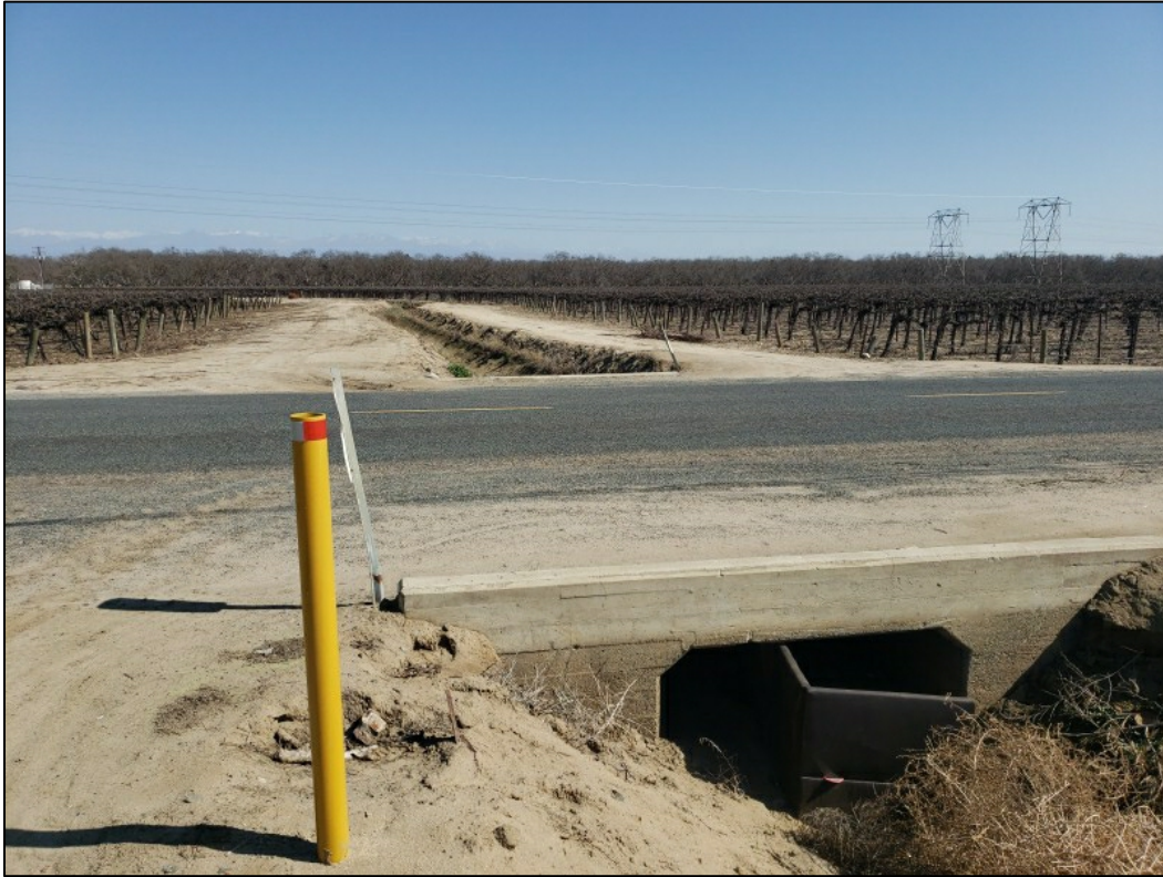
Figure 5. Segment of Extension Ditch passing beneath Road 148, looking west.
