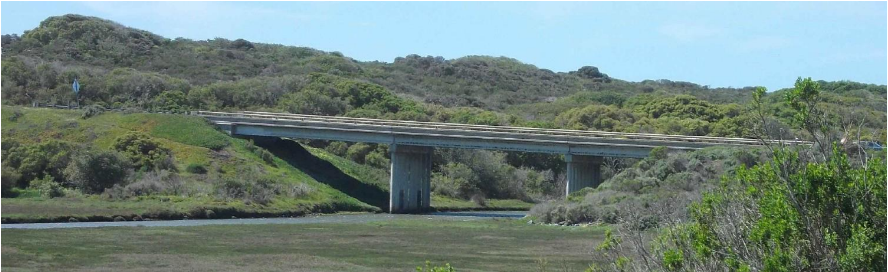
Figure 5a – Photo of existing bridge looking west
