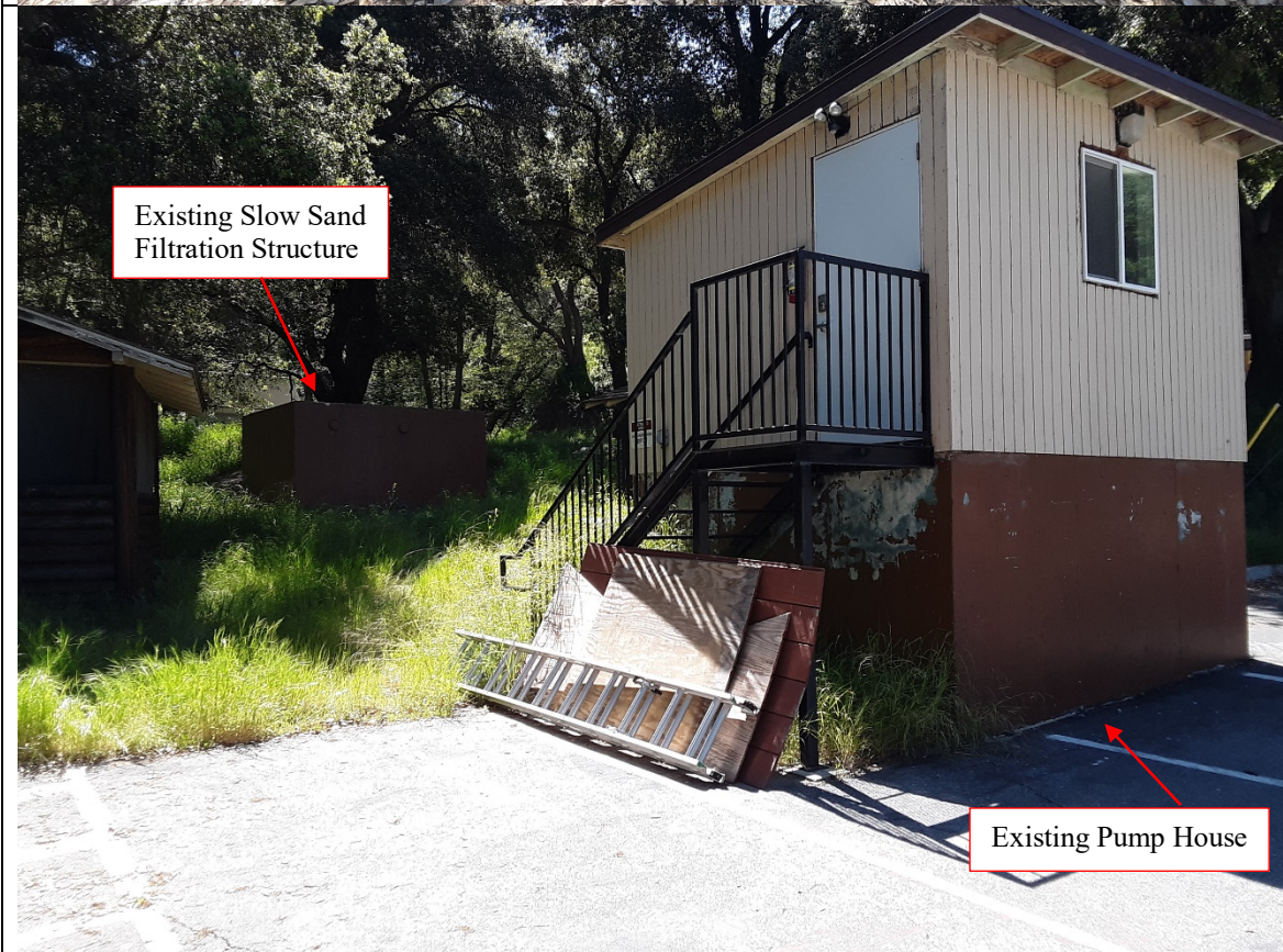
Photo 8. Looking SE at existing pump house and slow sand filtration structure.
