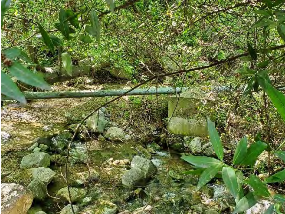
Figure 1. 4-inch pipe near concrete box structure
