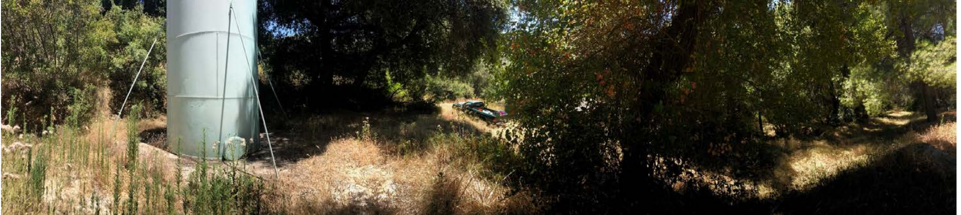
Photo 2: Panorama of existing reservoir
