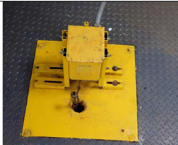
Figure 5. Floation sensor
