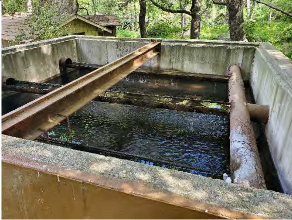
Figure 1. Slow sand filtration
