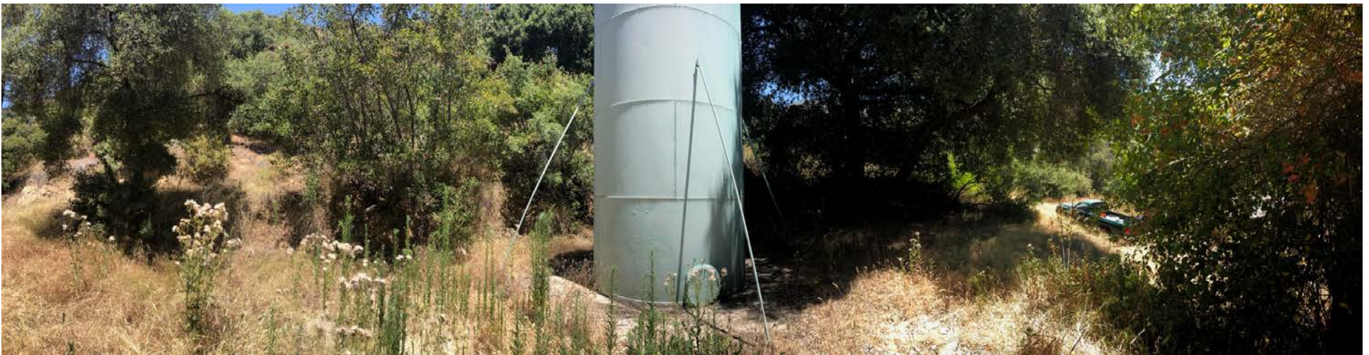
Photo 3: Panorama of existing reservoir
