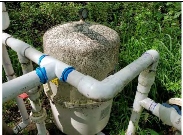
Figure 4. Diatomaceous filter from pretreatment system
