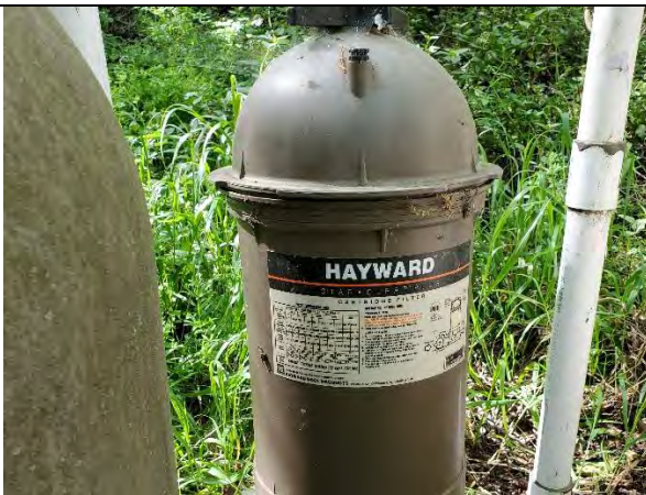
Figure 3. Cartridge filter from pretreatment system
