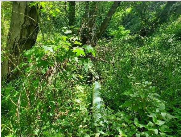
Figure 3. Steel pipe, east of pretreatment
