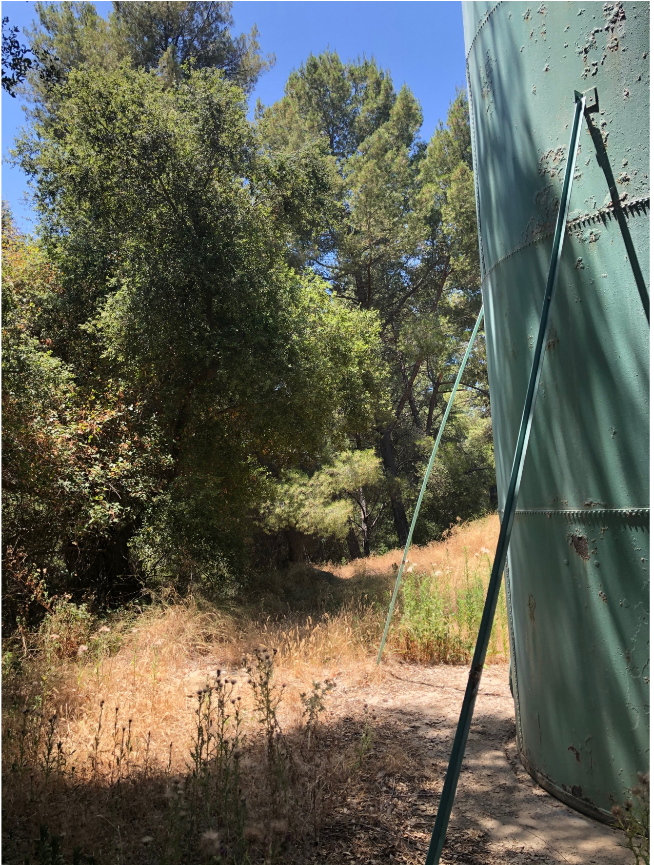
Photo 6: Existing reservoir and surrounding vegetation
