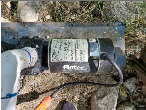
Figure 3. \frac{3}{4} HP Flotec pump
