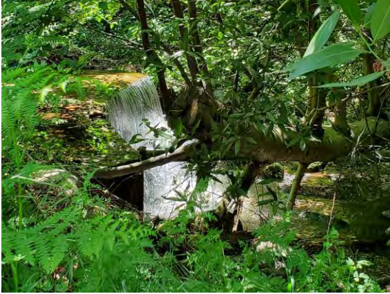
Figure 4-1. Concrete Box Structure
