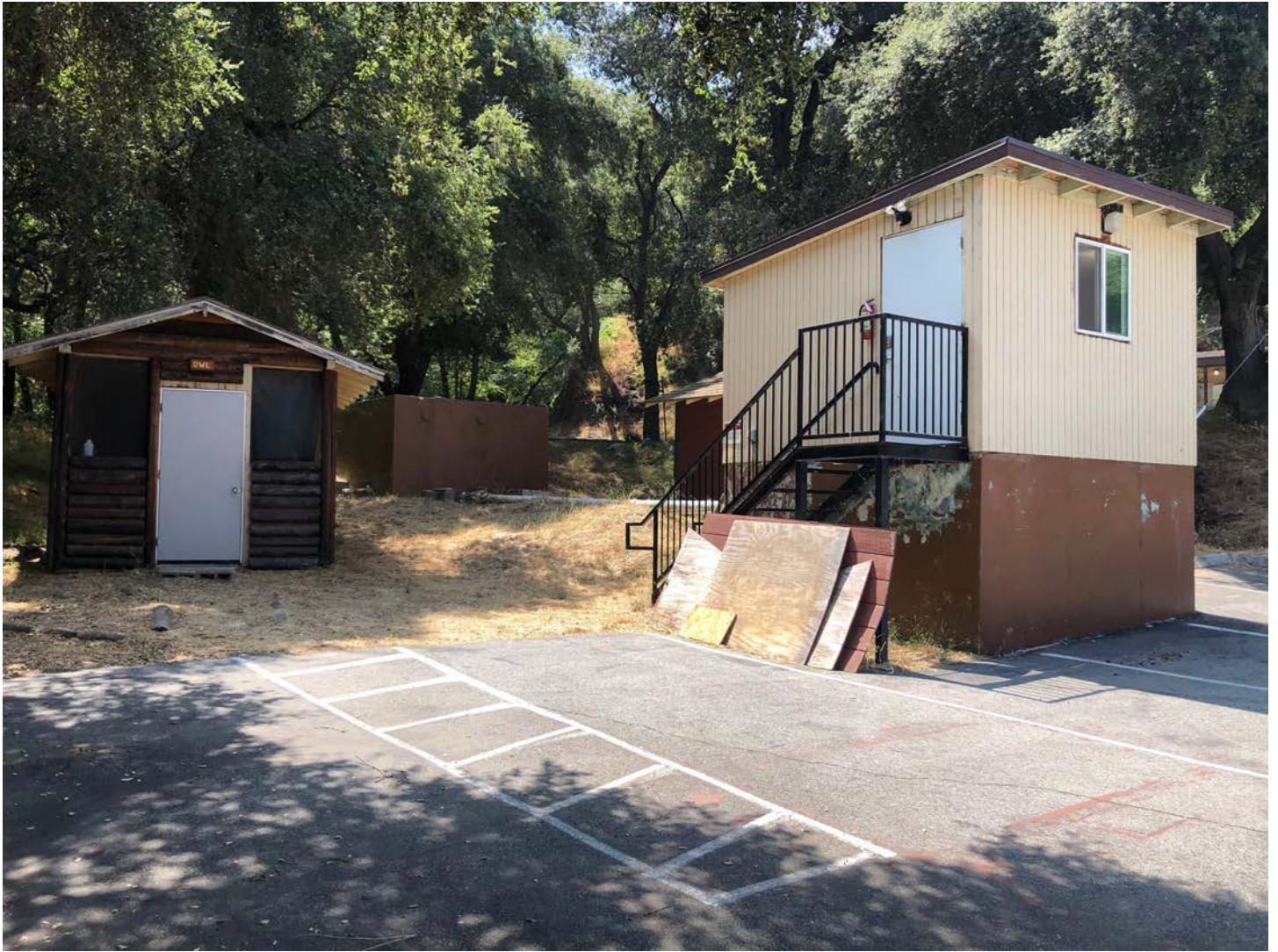
Photo 14: Pump house, pump station and clearwell viewed from lower Trask parking lot
