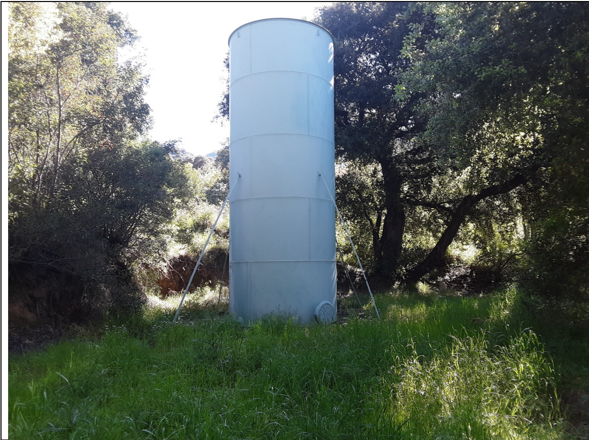
Photo 9. Looking E, at existing water storage reservoir (to be replaced).
