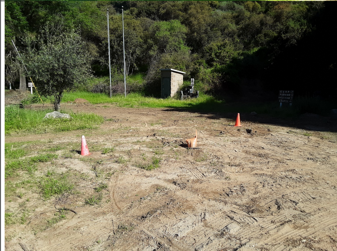
Photo 12. Potential new fire hydrant installation location.
