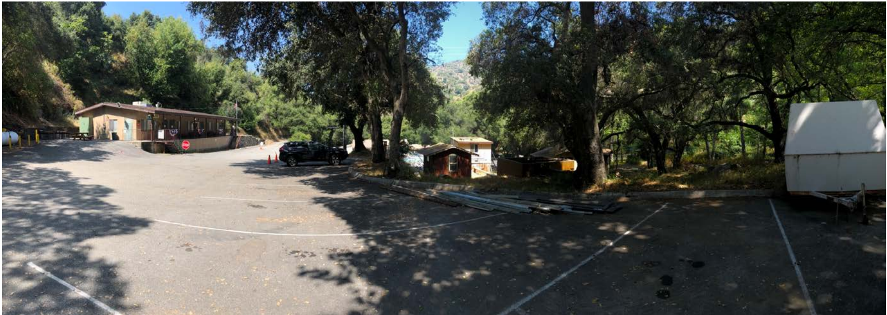
Photo 4: Panorama of parking area showing the slow sand filtration, pump house, pump station and clearwell housing
