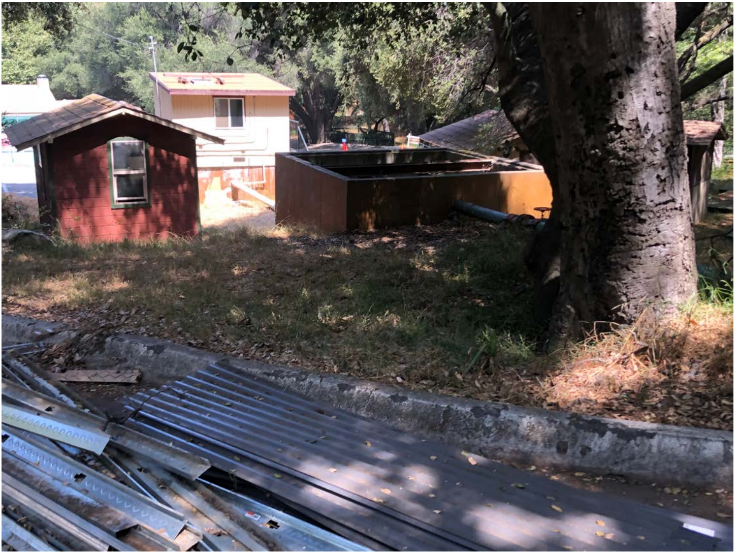
Photo 11: Existing slow sand filtration system and pump house, pump station and clearwell
