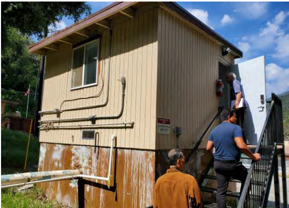
Figure 4-2. Clearwell / Pump House
