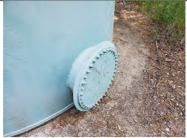
Figure 4. Discharge outlet
