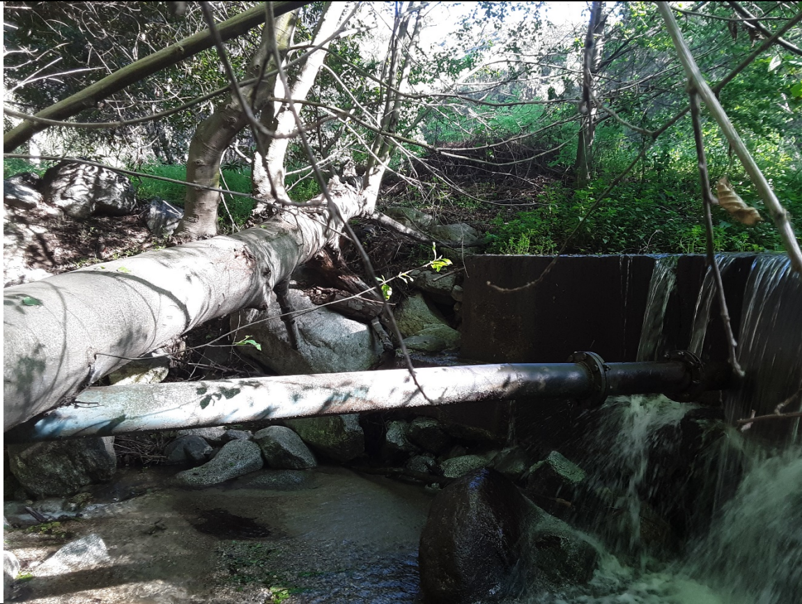
Photo 3. Remove fallen California bay tree ( Umbellularia californica ) over existing intake pipe.
