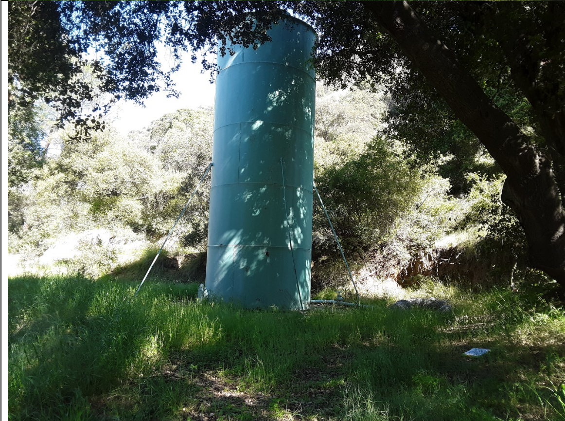
Photo 10. Looking NW, at existing water storage reservoir (to be replaced).
