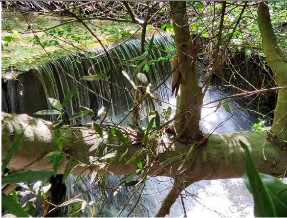
Figure 1. Concrete box structure
