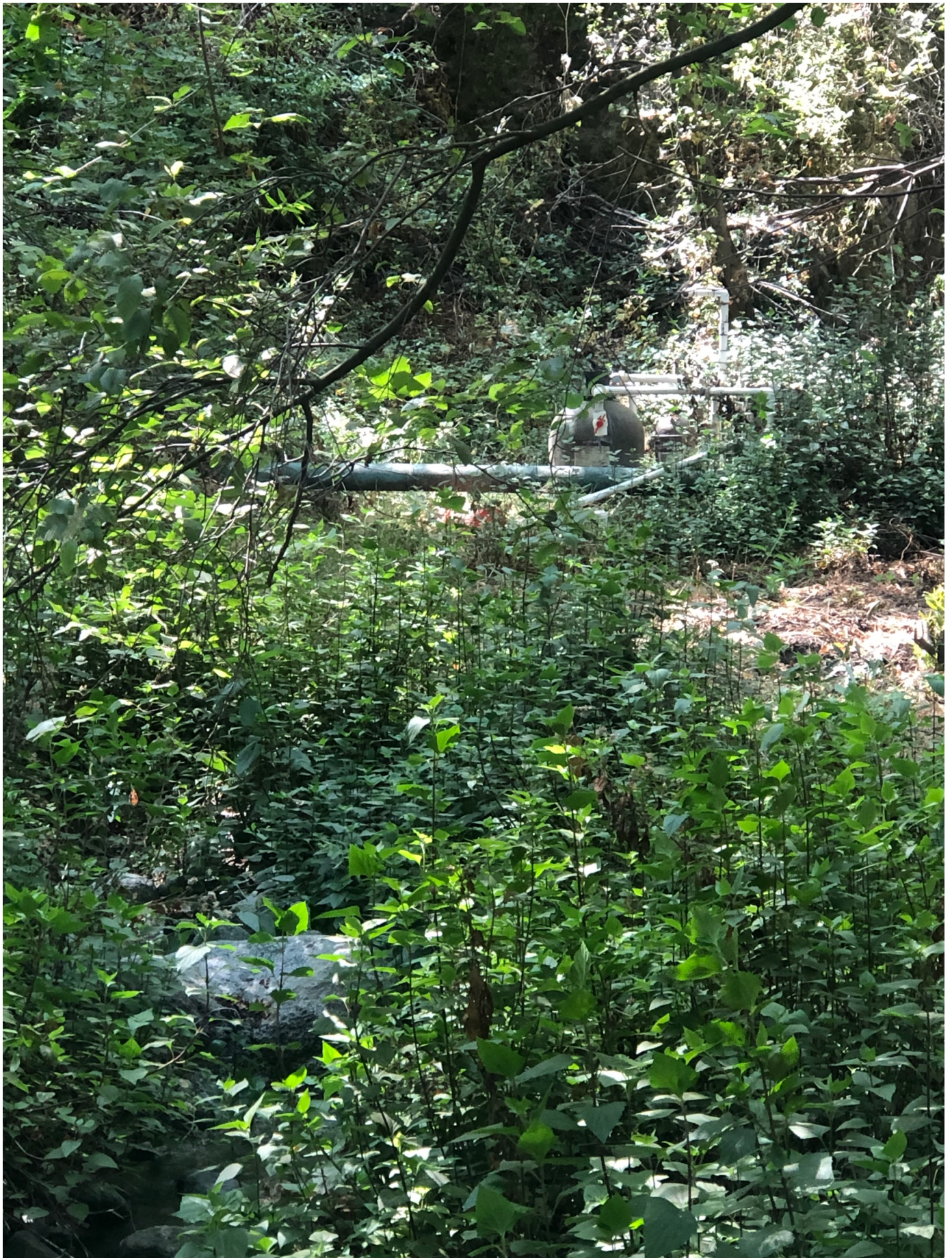
Photo 8: Existing reservoir and surrounding vegetation
