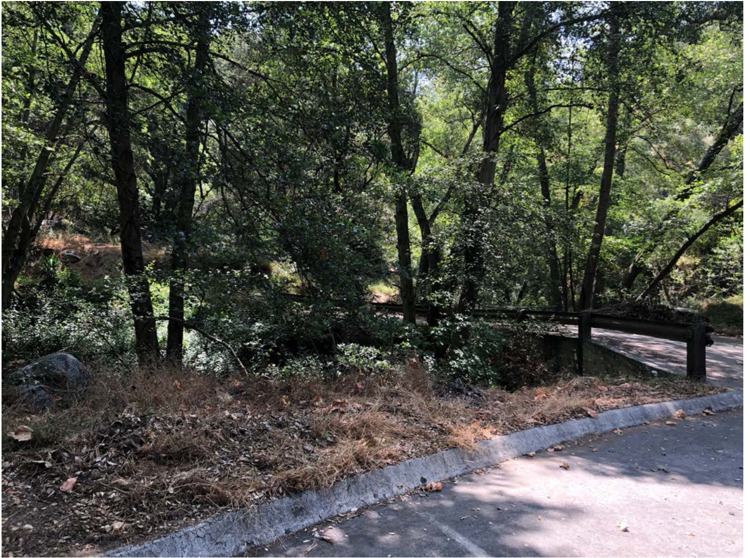
Photo 12: Trask parking lot pathway over sawpit wash near intake pipeline
