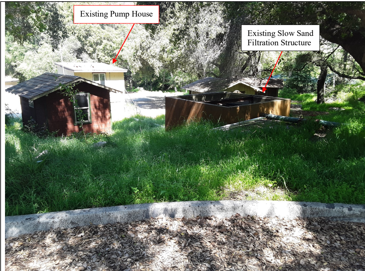
Photo 7. Looking NW at existing slow sand filtration structure and pump house. Slow sand filtration structure to be modified into a clear well with a pump station.
