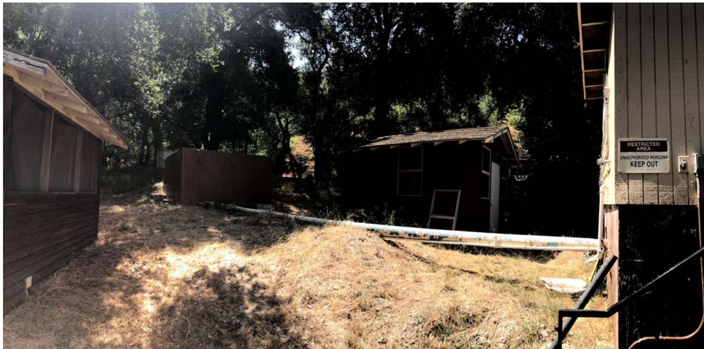
Photo 5: Photo showing the slow sand filtration and transmission to the pump house, pump station and clearwell housing
