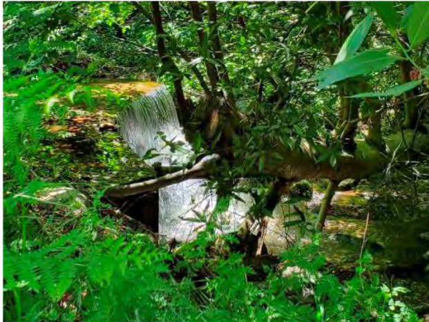
Photo 3: Concrete Box Structure
