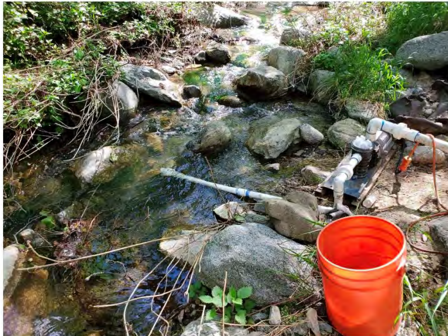
Photo 1: Sawpit Creek and Existing Temporary Collection Point
