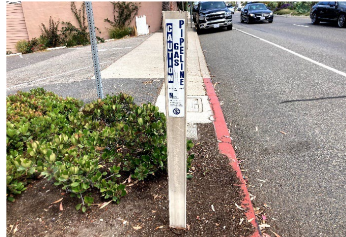
Photograph 4. View of the gas pipeline marker located on the eastern corner of the project site along Coast Highway, facing northwest.
