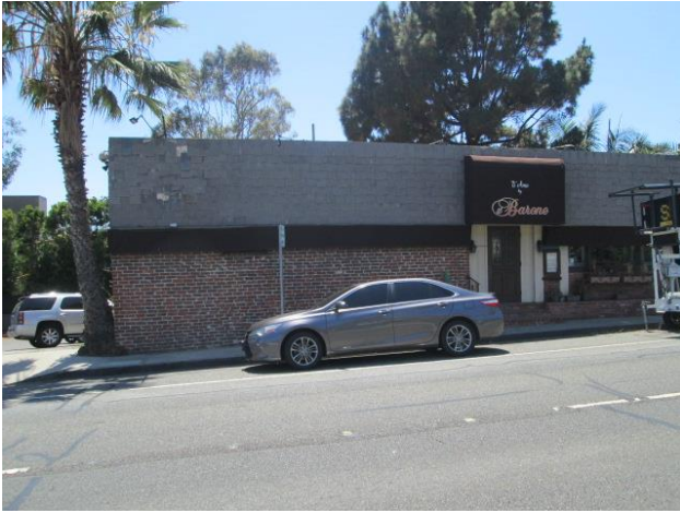
1. View of the northern portion of the Site from the east.
