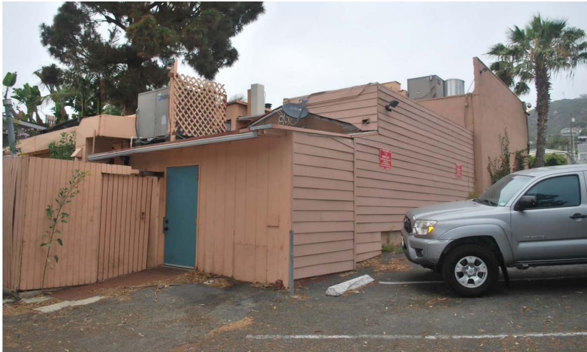
Altered rear section of 31727 Coast Highway, south and west elevations. Camera facing northeast.
