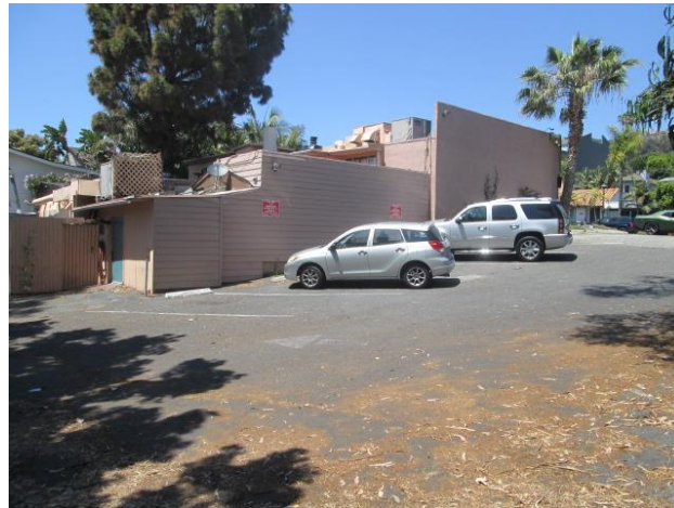
5. View of the Site from the south.
