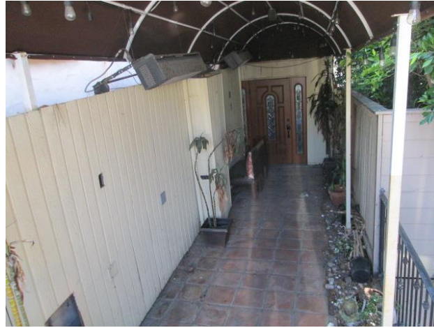
2. View of the entrance of the Site building.
