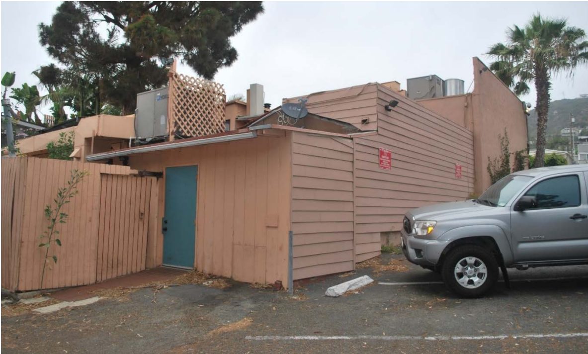
Figure 8 31727 Coast Highway, Rear Additions, Facing Northeast
