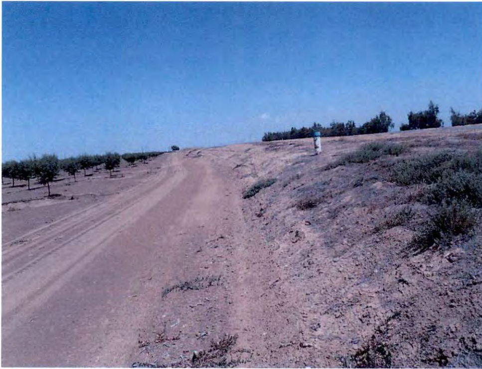
MP 139.27—Habitat facing upstream of an embankment that will be raised.
