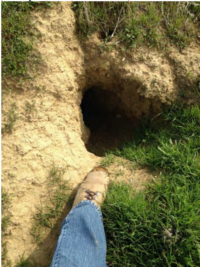
MP 137.60R - Burrow with sign on agricultural side of embankment (January 17, 2017, Laura Castro).
