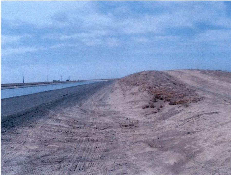
MP 137.30—Habitat facing downstream at an embankment that will be raised.
