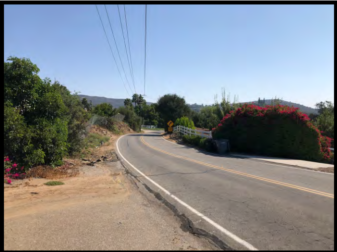
Photo #23: View looking east from main entrance.
