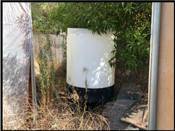
Photo #6: View of water tank along east side of greenhouses.
