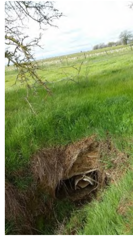
Photograph 2: Pipe located along west side of Subject Property, facing west.
