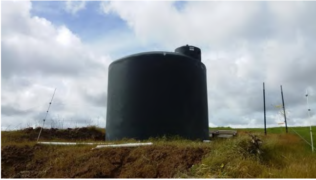
Photograph 9: 2,500 gallon AST by water well on east side of the Subject Property, facing south.
