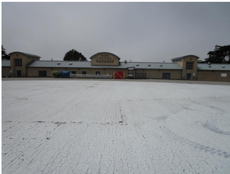
Figure 2. East elevation, looking west (IMG_0477)
