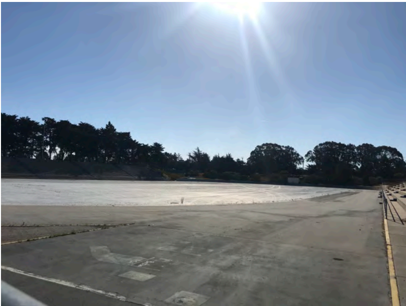
Interior project site looking northeast.
