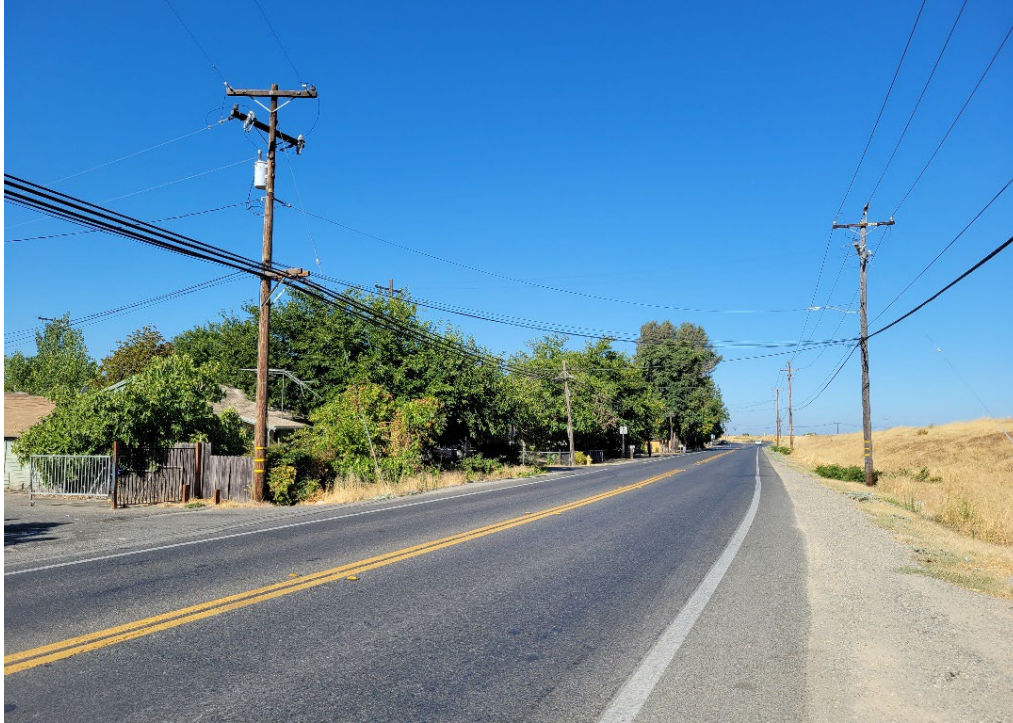
Figure 3.2-4. KOP-3: Yuba River South Levee Cutoff Wall Area, Facing West on Hammonton-Smartville Road (July 21, 2021).
