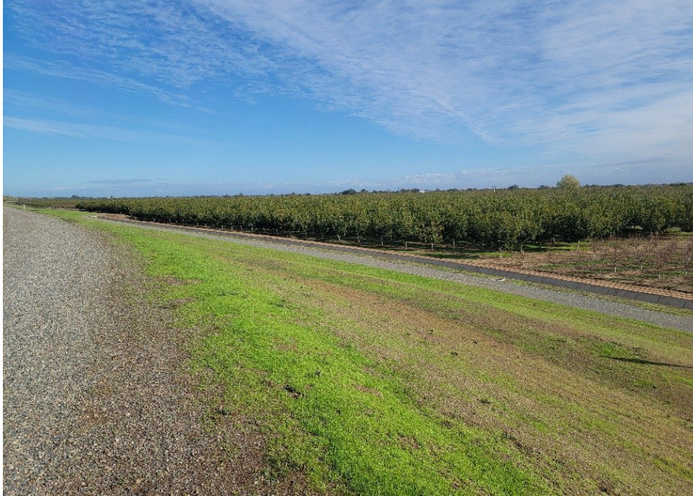
Figure 3.2-6. KOP-5: Feather River East Levee Seepage Remediation Area and Existing Relief Well System, Facing North (July 21, 2021).
