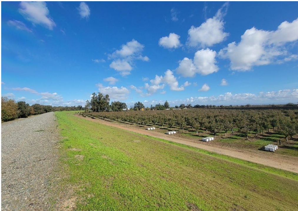
Figure 3.2-5. KOP-4: Feather River East Levee Raise Area, Facing North Toward Nearby Rural Residence (July 21, 2021).
