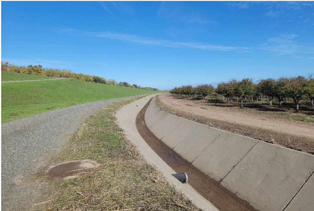
Figure 2-10. Relief Well and Drainage System along Feather River East Levee
