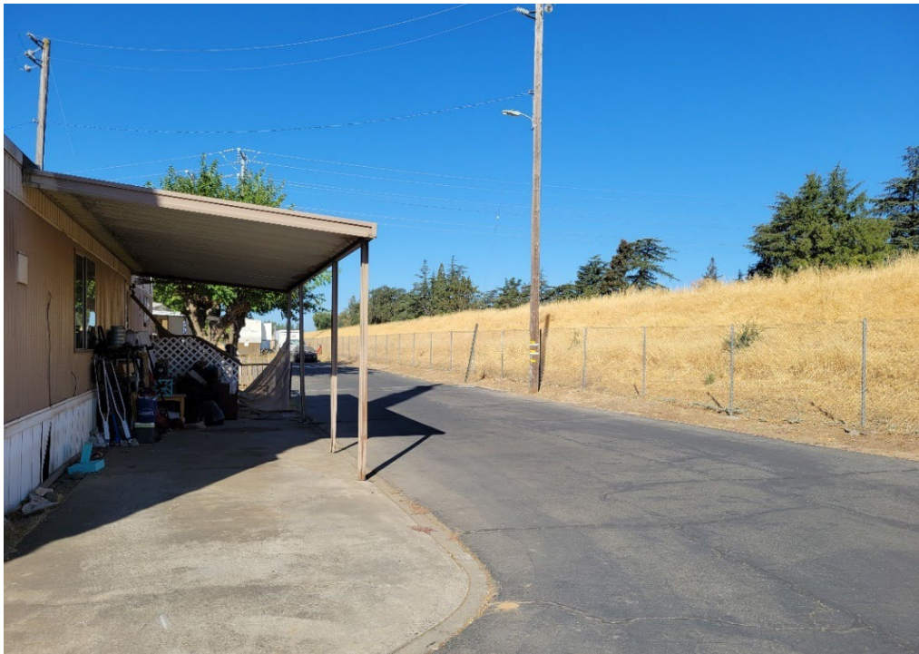
Figure 3.2-3. KOP-2: Yuba River South Levee Cutoff Wall Area, from Casa Mia Trailer Park, Facing West (July 21, 2021).
