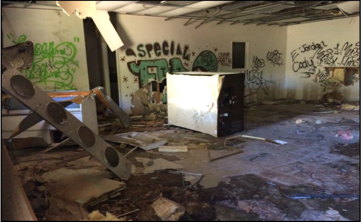
Photo 3. Interior of vacant building.
