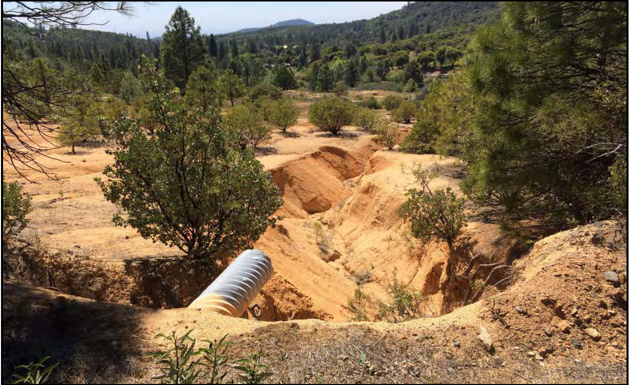
Photo 9. View of drainage culvert and erosional area within the Project Site.
