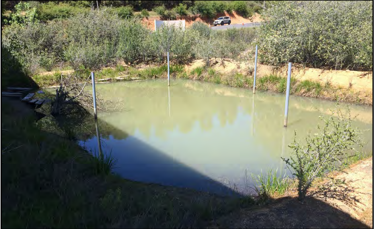
Photo 4. View of UST setting.
