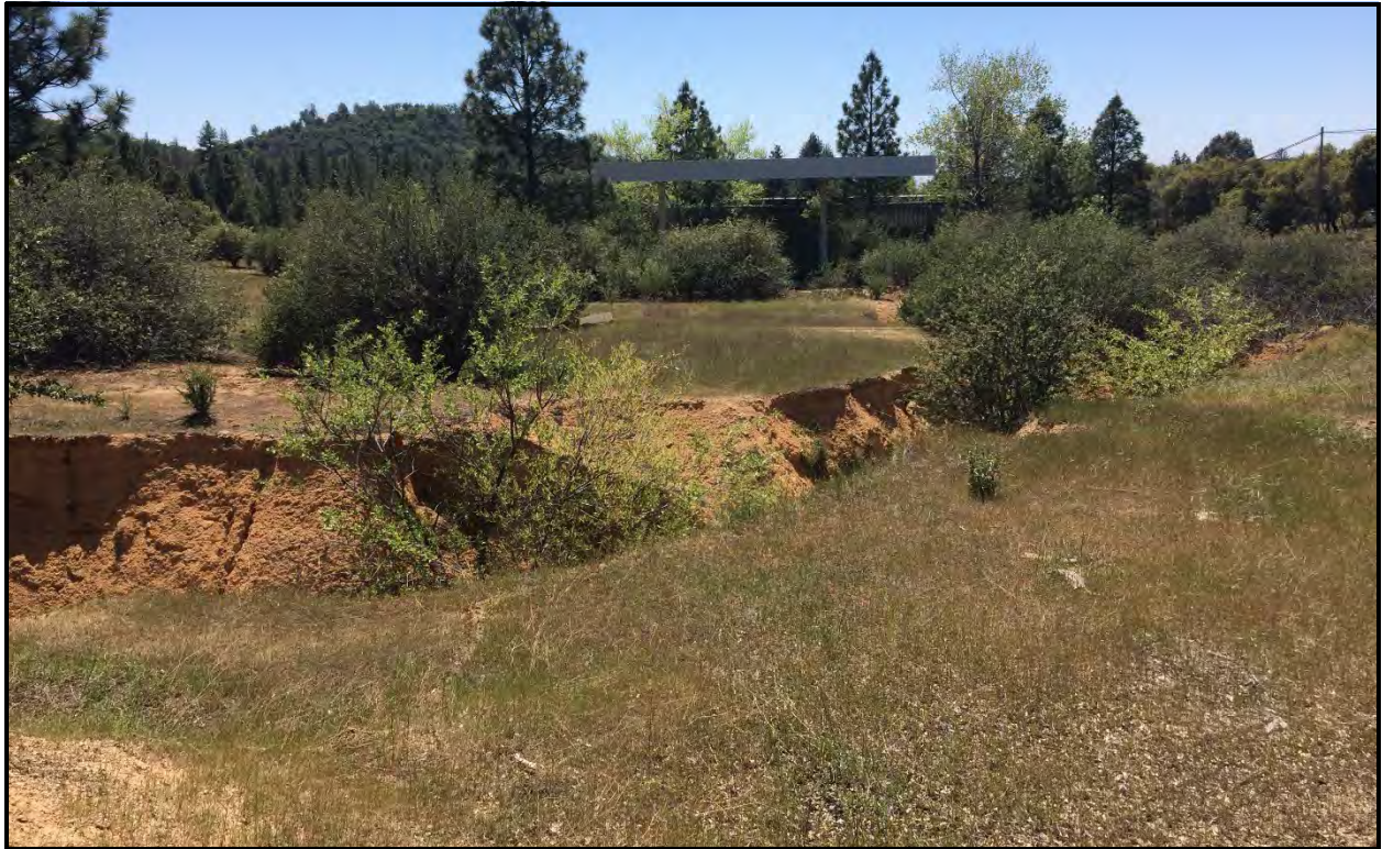
Photo 1. View of Former Service Station from Highway 120.
