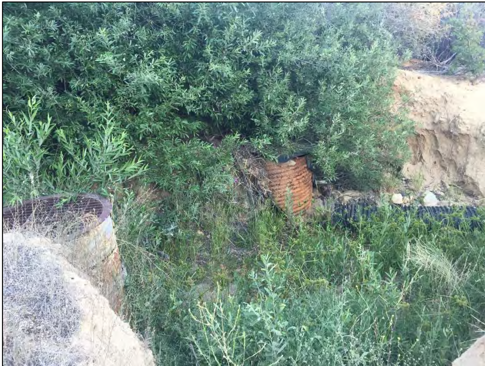
Photo 7. Intermittent channel and seep; standpipe (aspect south; 7/21/20).
