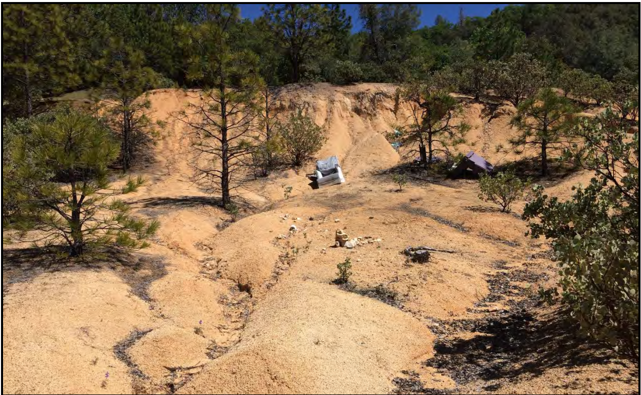
Photo 8. Southern portion of Project Site.
