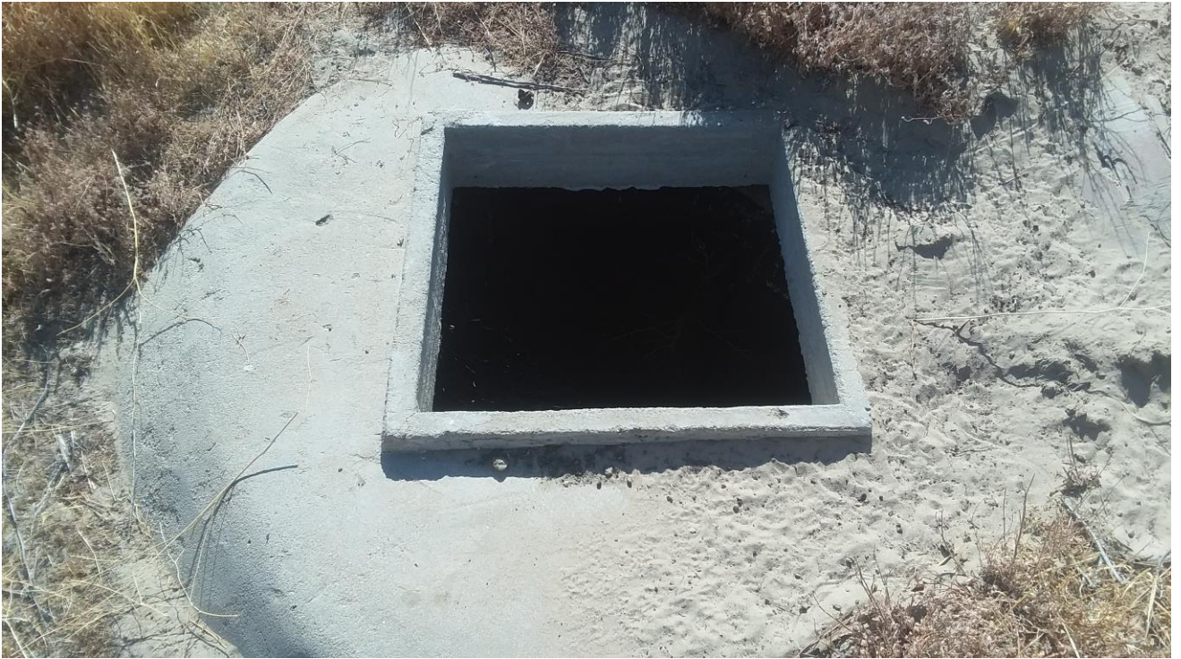
Figure 6 Site R-3, Underground Cistern
