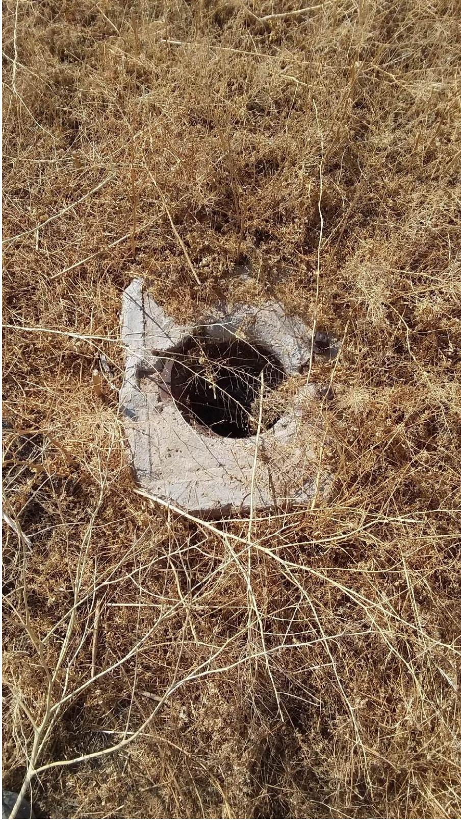
Figure 4 R-2, Underground Waterline
