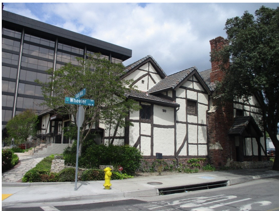
Figure 20. 100 N Santa Anita Avenue: side (south) and primary (west) elevation, view looking northeast (IMG 6349)
