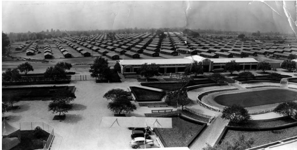
Figure 5. Barracks to house Japanese internees at the Santa Anita Park Racetrack, 1942 (Los Angeles Public Library)
