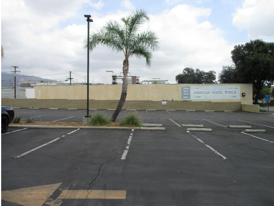
Figure 18. 25 Wheeler Avenue: West side elevation, view looking east (IMG 6260)
