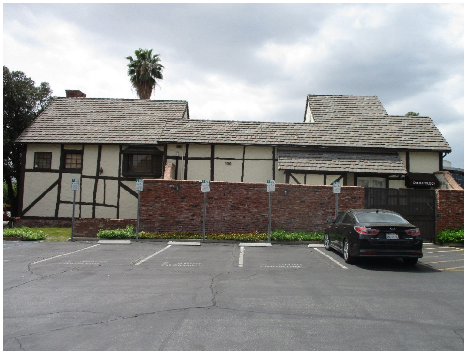
Figure 21. 100 N Santa Anita Avenue: rear (east) elevation, view looking west (IMG 6383)
