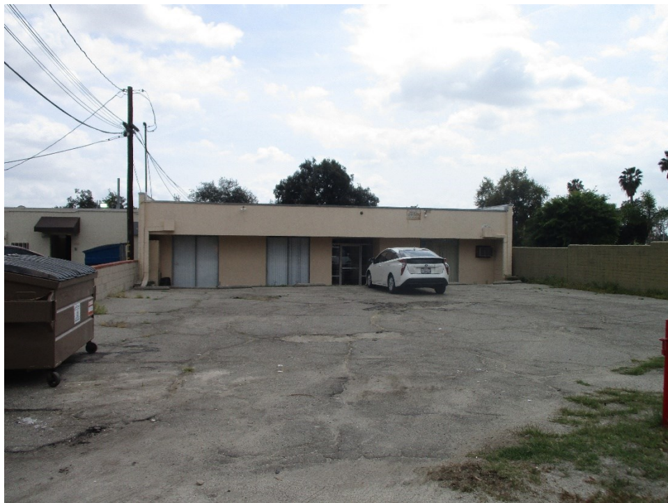
Figure 17. 25 Wheeler Avenue: Rear (north) elevation, view looking south (IMG 6291)
