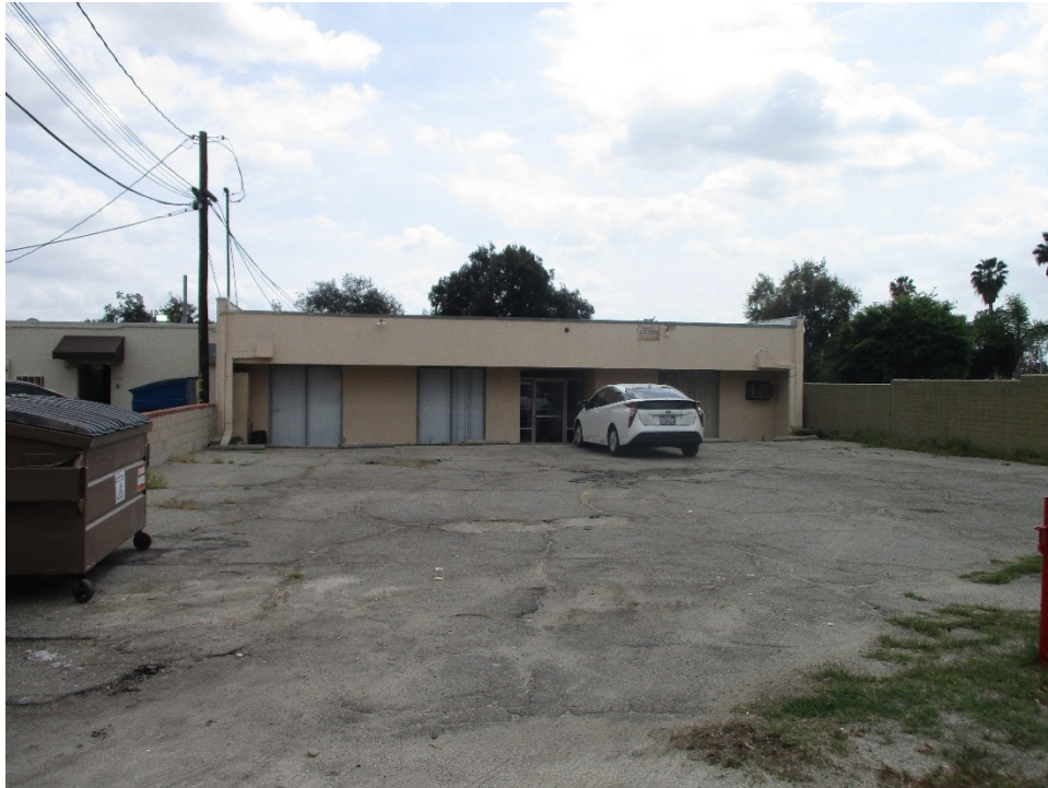
Figure 2. 25 Wheeler Avenue: Rear (north) elevation, view looking south (IMG 6291)
