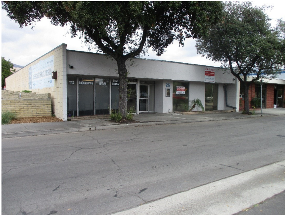
Figure 1. 25 Wheeler Avenue: primary (south) and west elevation, view looking northeast (IMG 6264)
