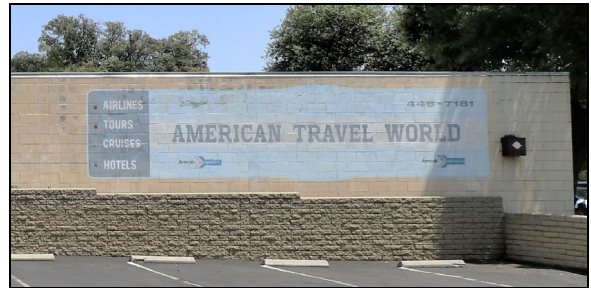
West elevation (southern end), view to the east (5/7/21). Painted, non-historic wall sign.
