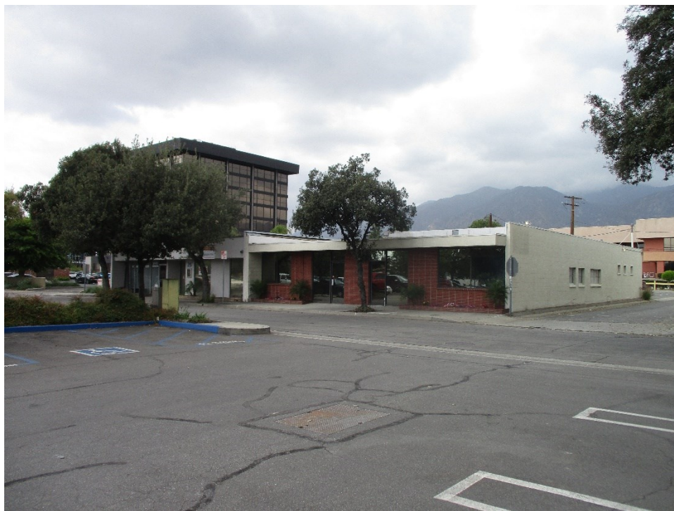
Figure 13. 31-33 Wheeler Avenue: primary (south) and east elevation, view looking northwest; 25 Wheeler Avenue and 150 N Santa Anita Avenue in background(IMG 6274)
