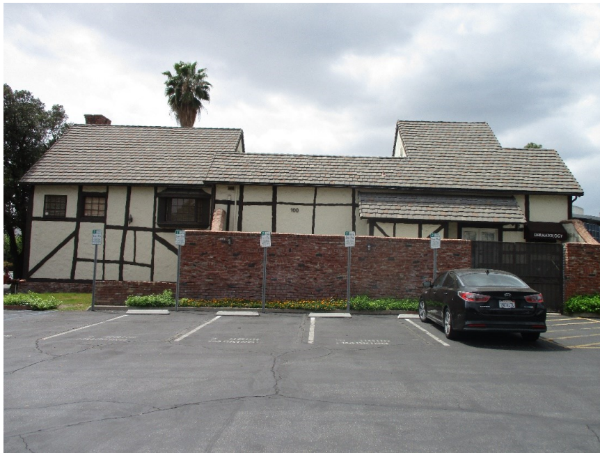
Figure 2. 100 N Santa Anita Avenue: rear (east) elevation, view looking west (IMG 6383)
