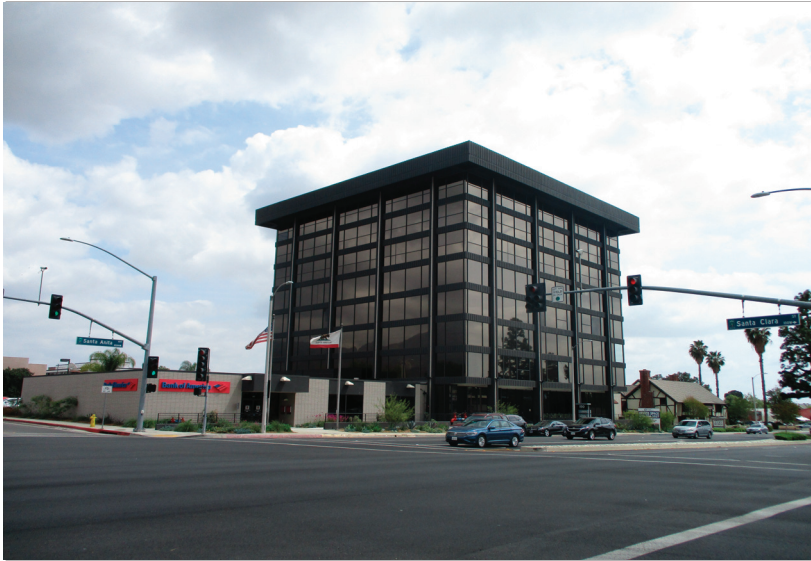
Photo 1: Southwestern view of the single-story bank, eight-story office building, and off-site commercial building from the northwest corner of N. Santa Anita Ave. and Santa Clara St.
