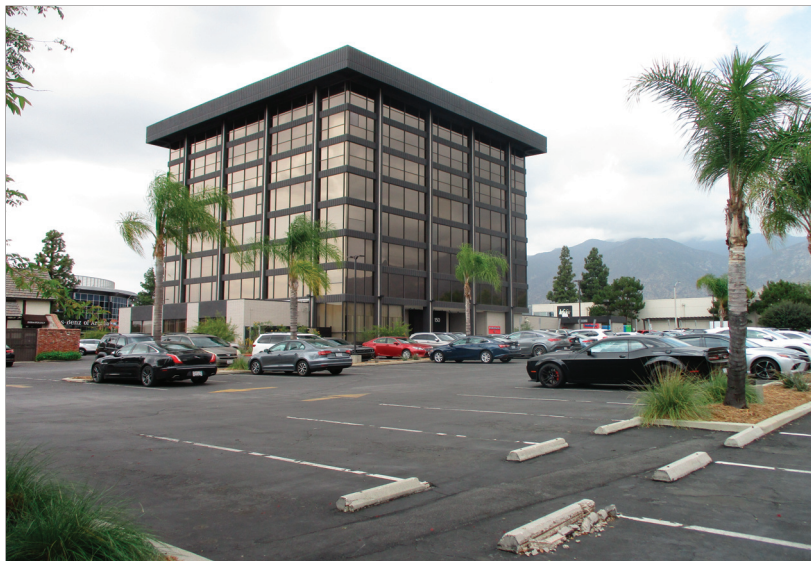
Photo 6: Northwestern view of the main parking lot and backside of the eight-story office building.
