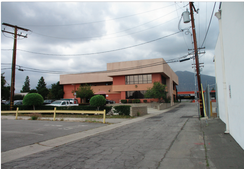
Photo 3: Northwestern view of the off-site and on-site alleys, as well as the backside of the two-story commercial building from the off-site alley.
