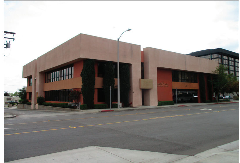
Photo 2: Southwestern view of the two-story commercial building from the north side of Santa Clara St.
