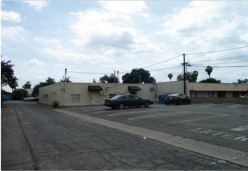
Photo 4: Southwestern view of the two single-story office buildings from the off-site alley.
