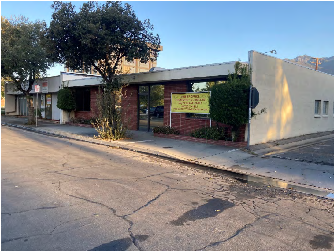
View of front of 33 Wheeler Ave building
