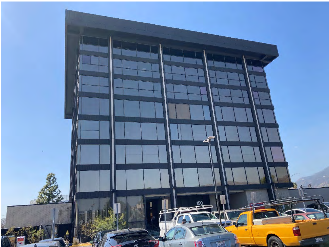
View of east side of 150 N. Santa Anita Ave building
