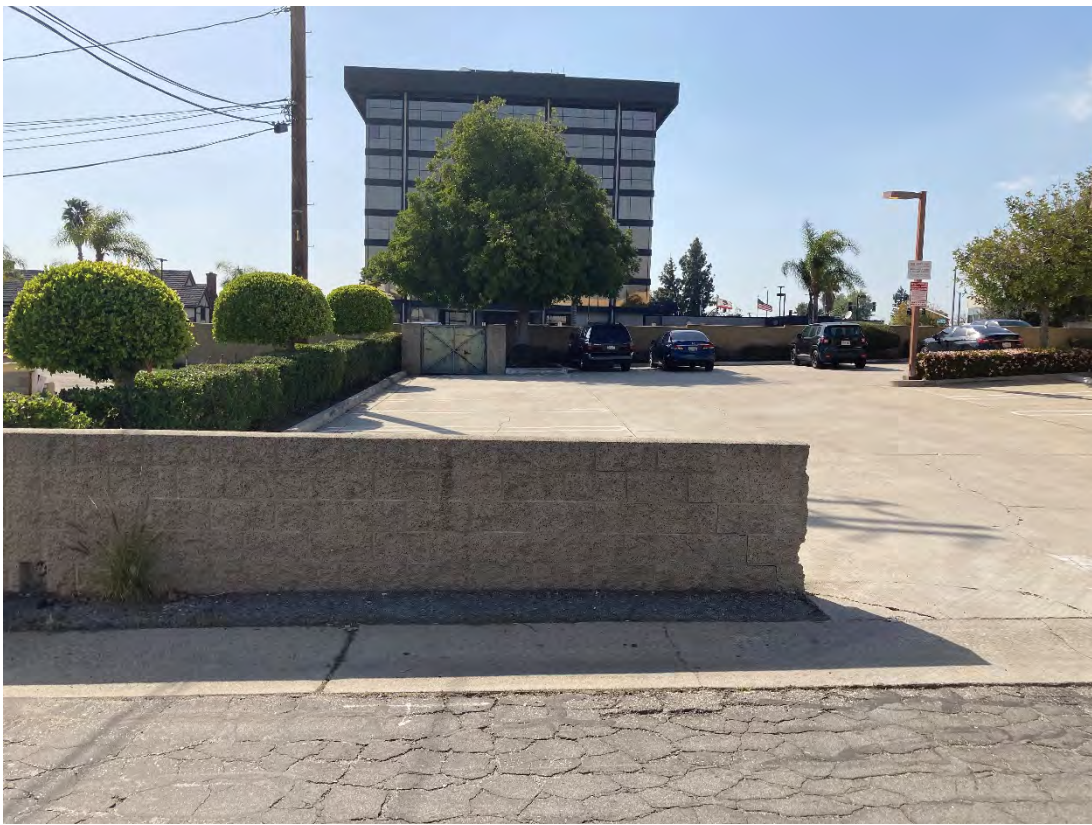
View of typical parking lot / exterior portions of Site located south of 30 E. Santa Clara St
