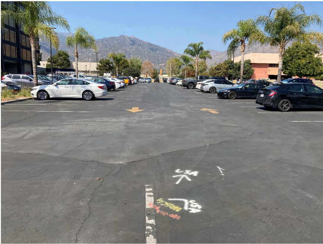
View of typical parking lot / exterior portions of Site located south and east of 150/180 N. Santa Anita Ave
