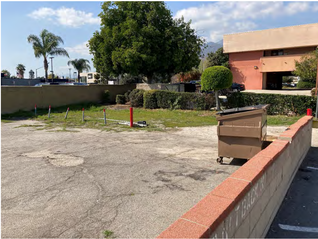
View of typical parking lot / exterior portions of Site located north of 25 Wheeler Ave
