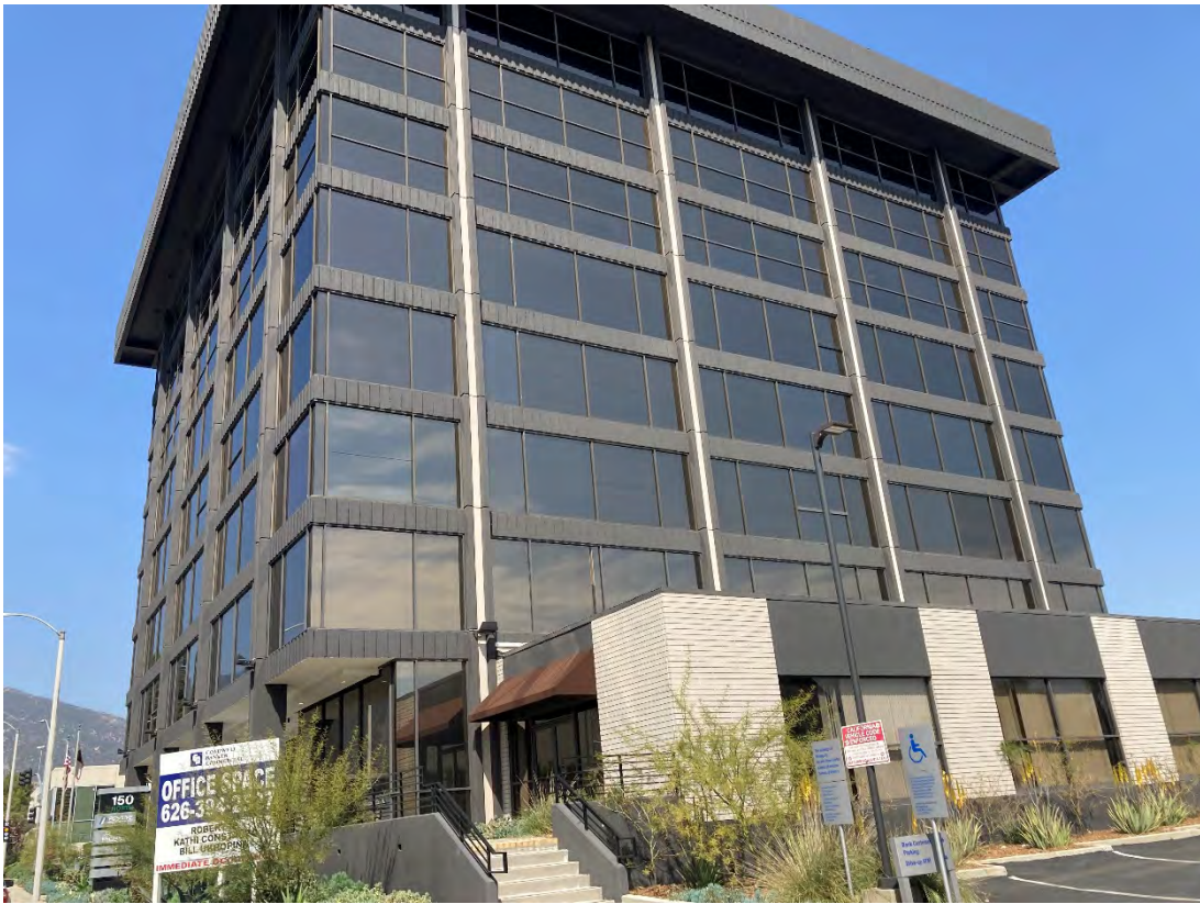
View of south side of 150 N. Santa Anita Ave building
