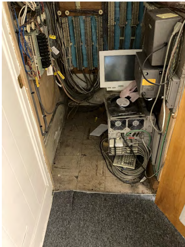
View of storage area / phone room in 33 Wheeler Ave
