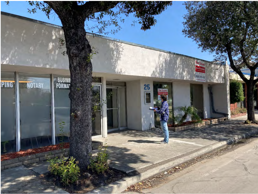
View of front of 25 Wheeler Ave building
