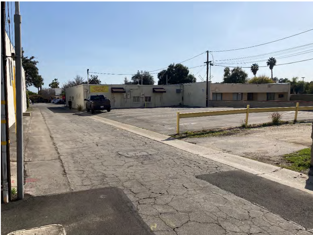
View of typical parking lot / exterior portions of Site located north of 33 Wheeler Ave
