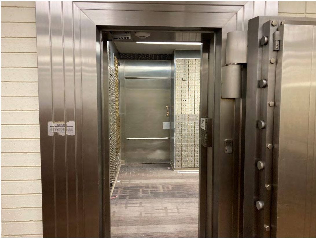
View of entrance to bank vault at 180 N. Santa Anita Ave
