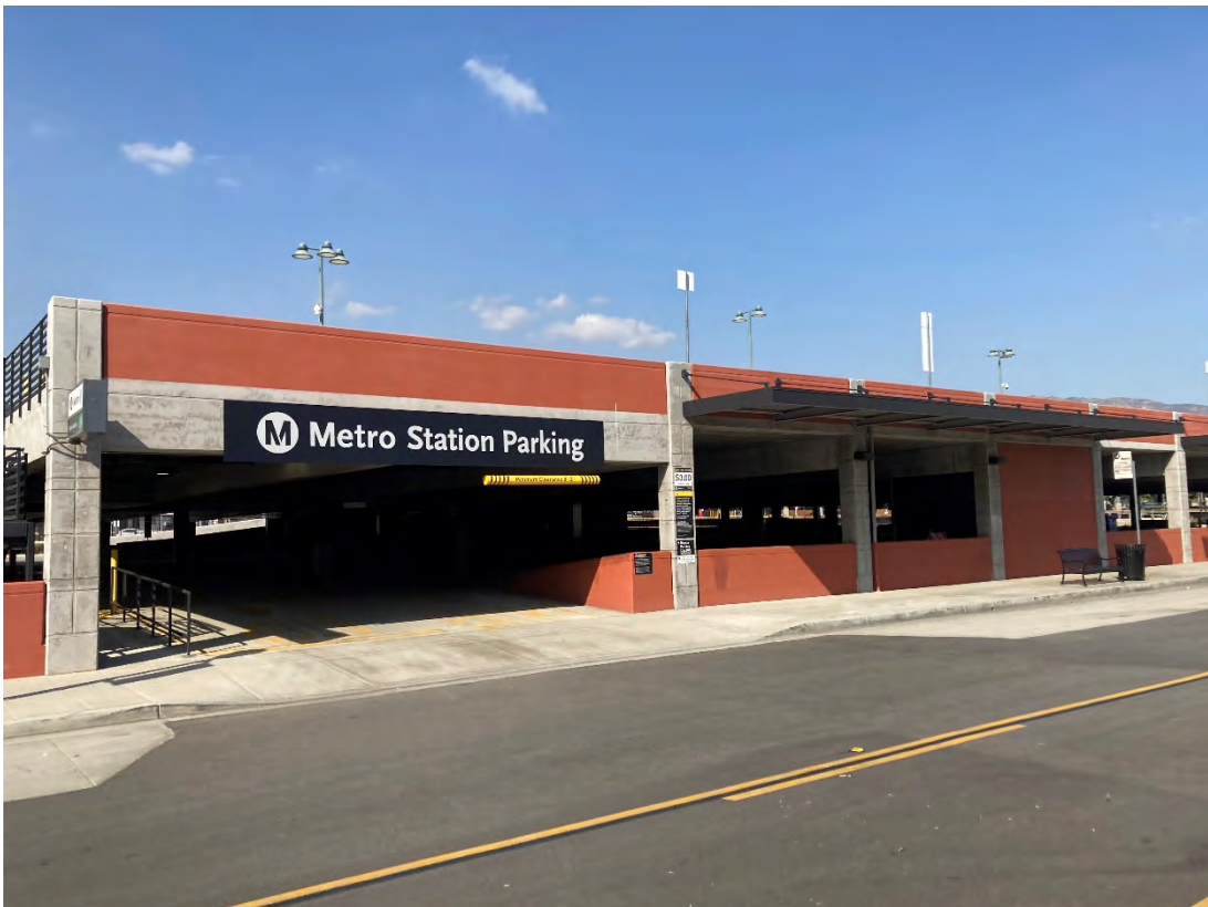
View of the parking structure located to the north of the Site across Santa Clara Ave
