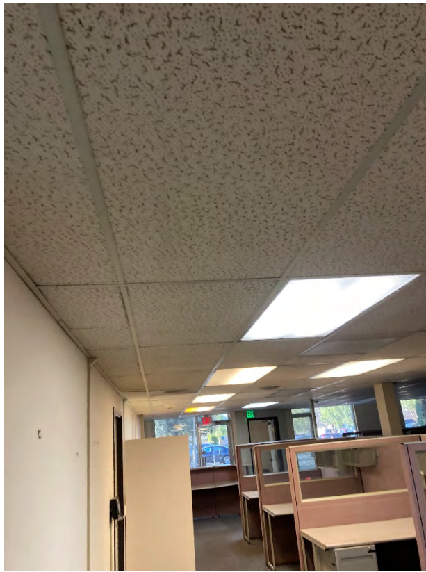
View of office space in 33 Wheeler Ave
