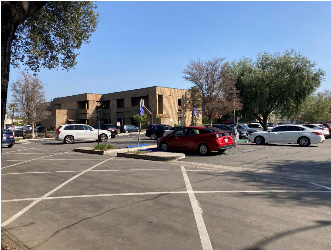
View of retail parking lot located to the south of the Site across Wheeler Ave
