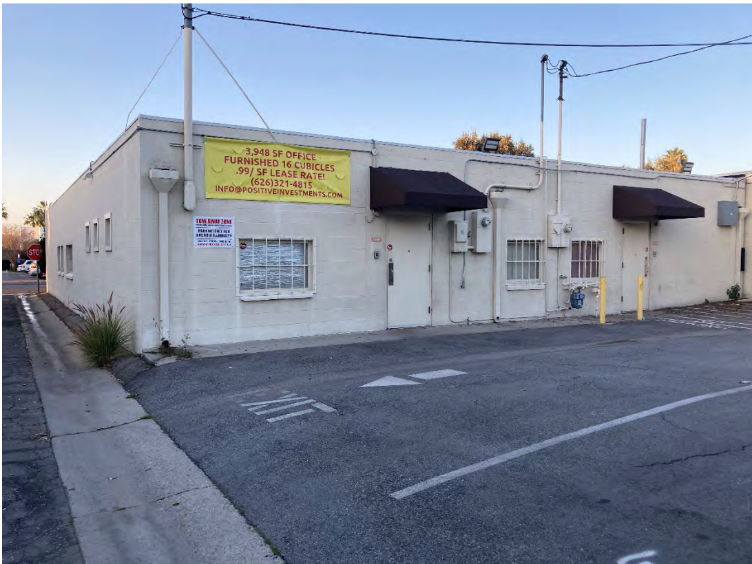
View of rear of 33 Wheeler Ave building
