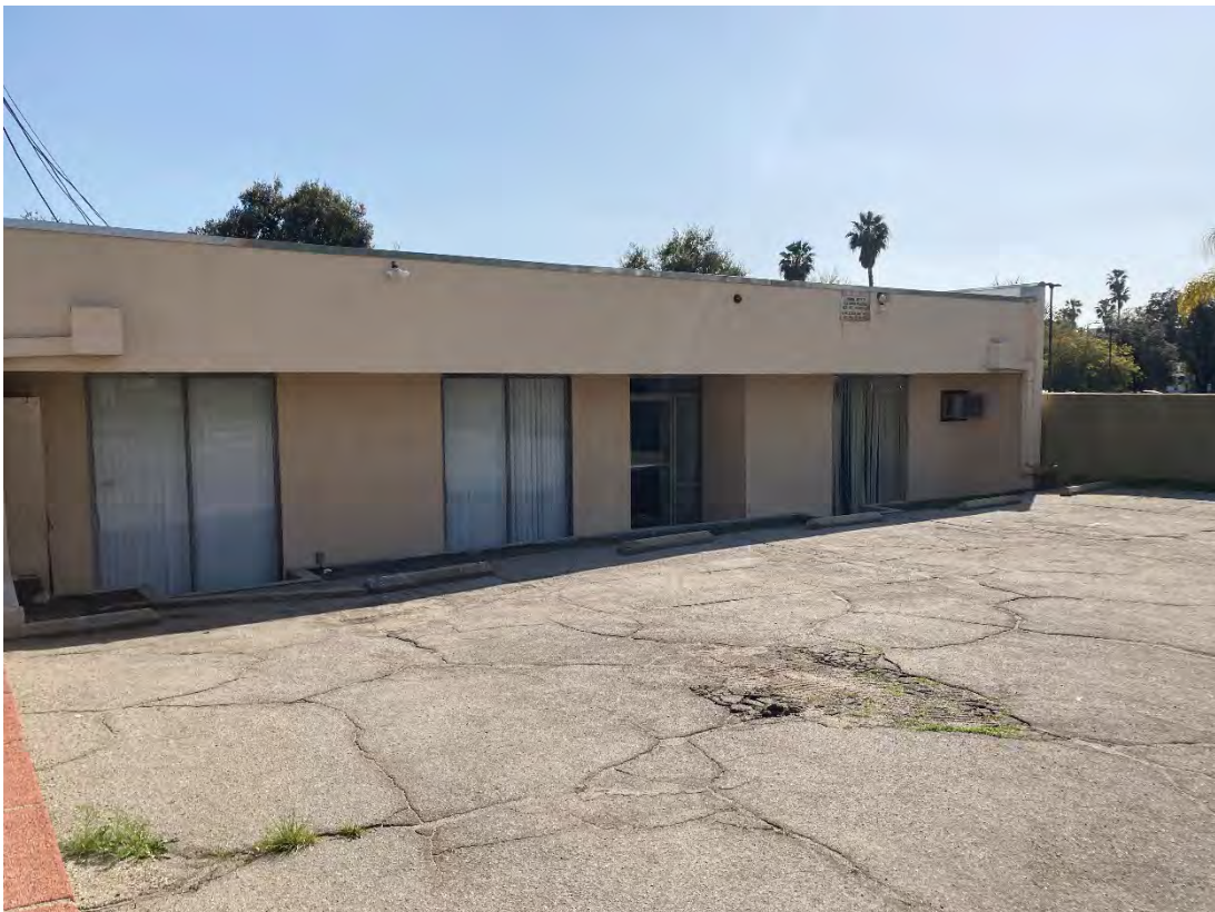
View of rear of 25 Wheeler Ave building
