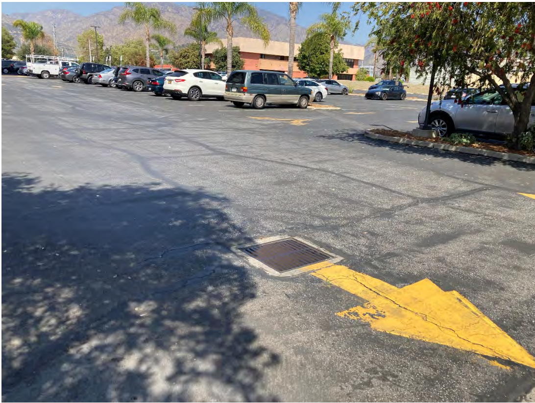
View of storm drain on south side of Parcel B (150/180 N. Santa Anita Ave)
