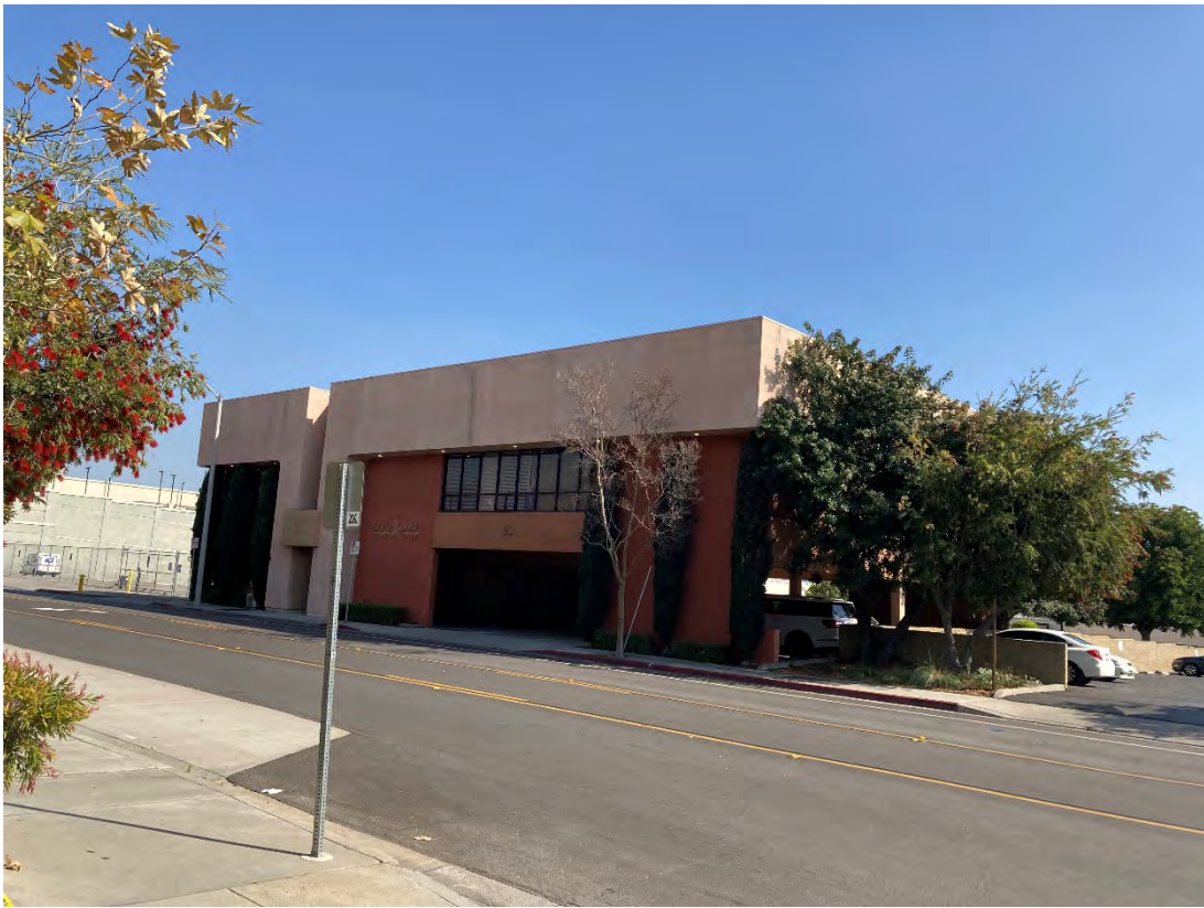
View of front of 30 E. Santa Clara St.
