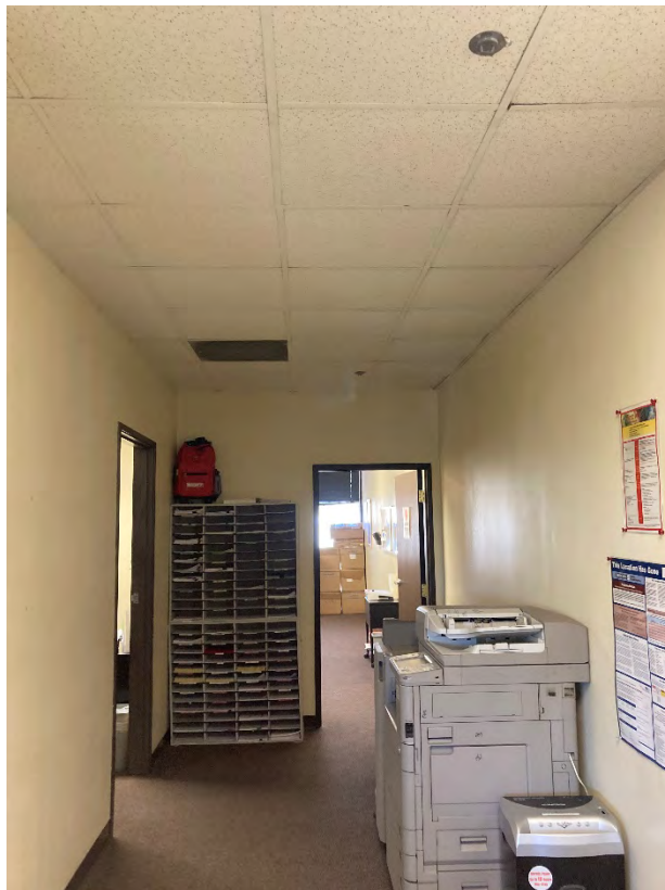
View of typical office space at 30 E. Santa Clara St
