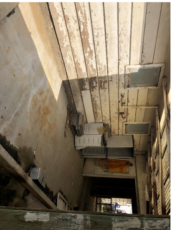
Photo 26: East side office building
