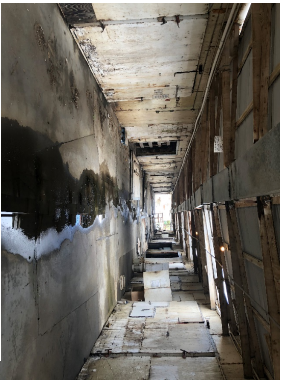
Photo 19: View to north southeast covered walkway
