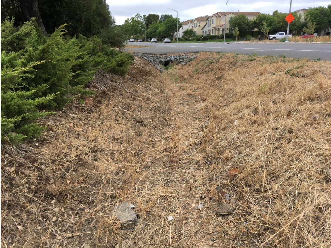
Photo 3. Roadside ditch along Watsonville Road looking southwest (Sample point 3).
