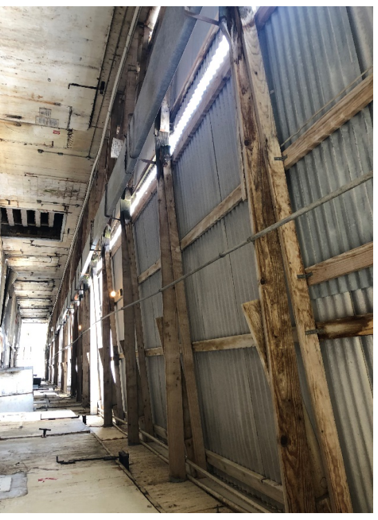
Photo 20: Galvanized roofing covered walkway
