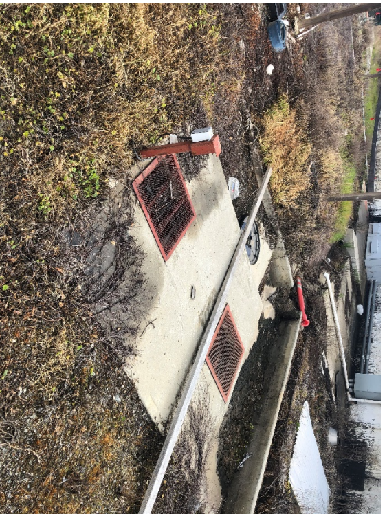
Photo 9: Rainwater sump south of office building
