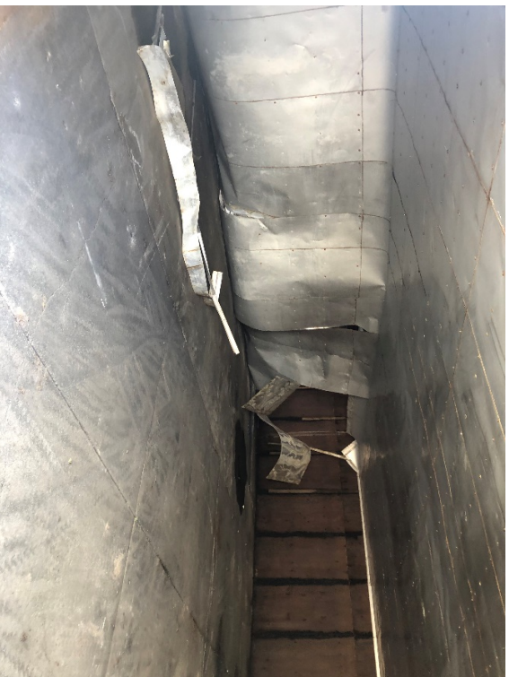
Photo 23: Northeast drying building interior
