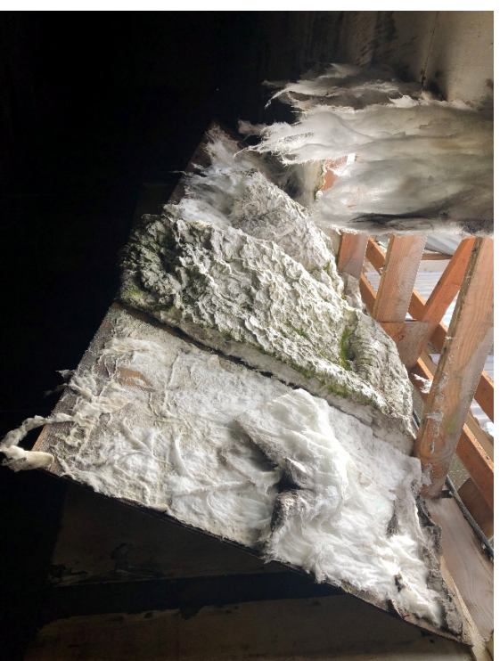
Photo 24: Northern drying building ceiling insulation
