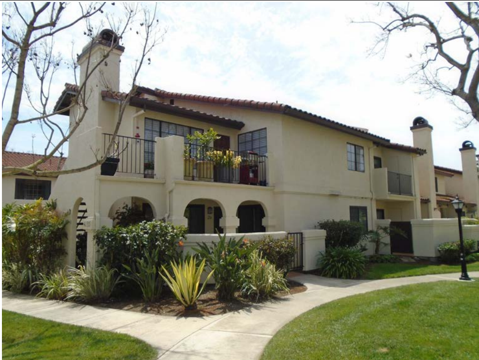
Figure 17. Example of a townhome development in La Jolla Colony, Las Palmas, Map ID #59 (DSC02403)
