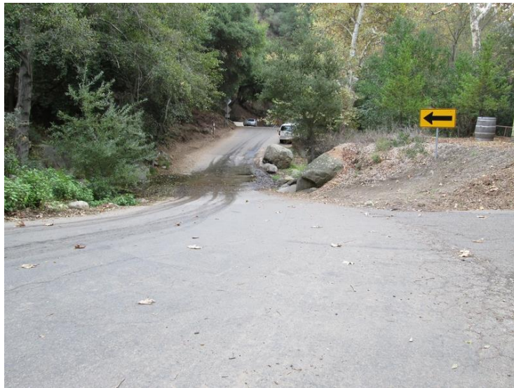
Photograph 2. Low Water Crossing Pre-TFDFI, September 2016 (view east)
