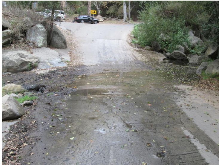
Photograph 1. Low Water Crossing Pre-TFDFI, September 2016 (view west)
