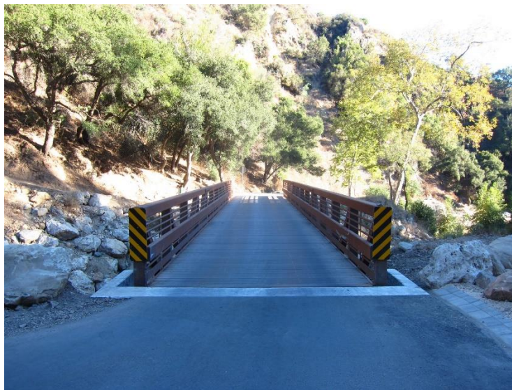
Photograph 5. Post-TFDFI Existing Condition with Temporary Bridge, December 2020 (view east)
