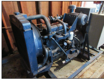
Figure 9. Generator repaired and operational
