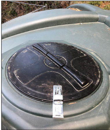
Figure 10: Roof lock on China Grade Tank.
