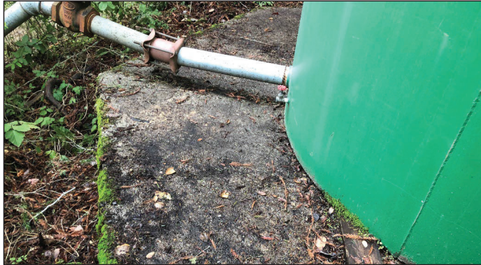
Figure 12: Oberst Station existing foundation
