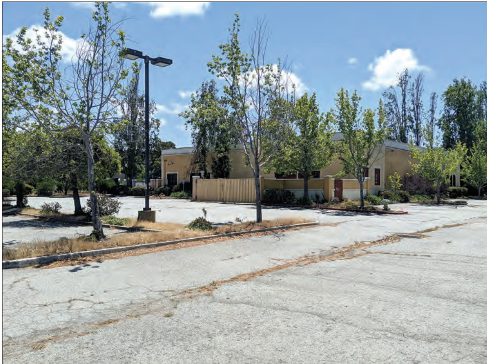
Photo 2: View from the northwest corner of the project site, looking southeast
