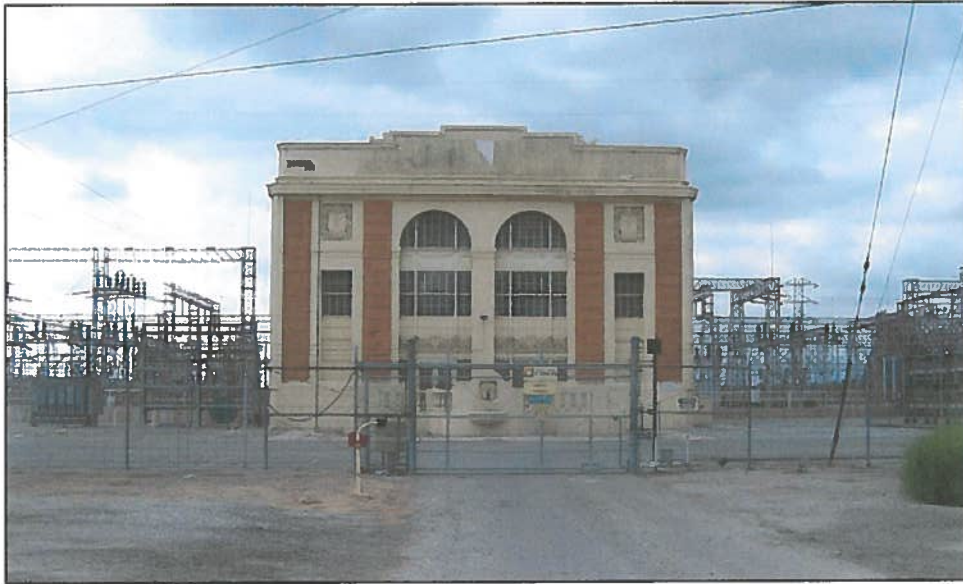
Photograph 4: Origination point of SSPC powerline discussed herein: this Edison substation is located west of the intersection of Chestnut and Grape in the City of San Bernardino near Mill Street. The building appears to be the original SSPC First Steam Plant, built in 1910-1911, and is in excellent condition. Note lion fountain behind entrance gate. Insets in upper right and left corners of the façade shown below. Other historic power lines emanate from this substation, as does the line north to the Owens Valley. The switching yard exhibits towers and steel frameworks many of which were likely built more than 45 years ago.
