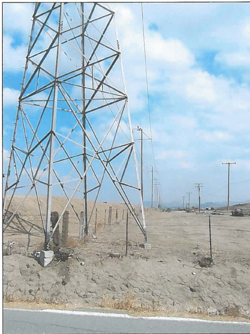
Photograph 1: View of a tower at the northeast corner of the Edgewater property along Cucamonga Road in south Chino, San Bernardino County. View due east. Another steel tower can be seen in the distance.
