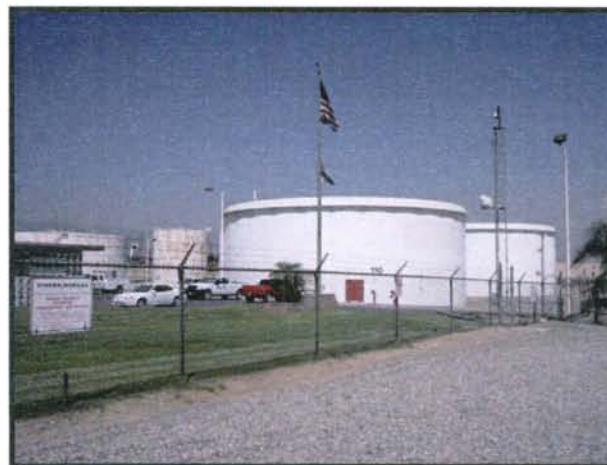
View to the East-Northeast. Note infill construction of new tanks in foreground
