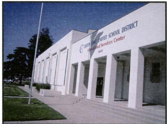
View to the North
