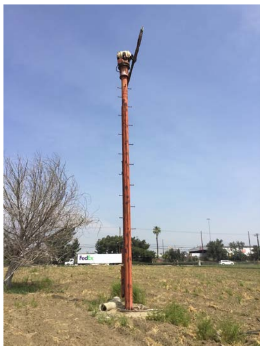
Photograph 5: Close-up of Windmill 2.
