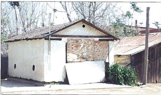
Garage, western and southern elevations, view to the northeast (3/23/15).
