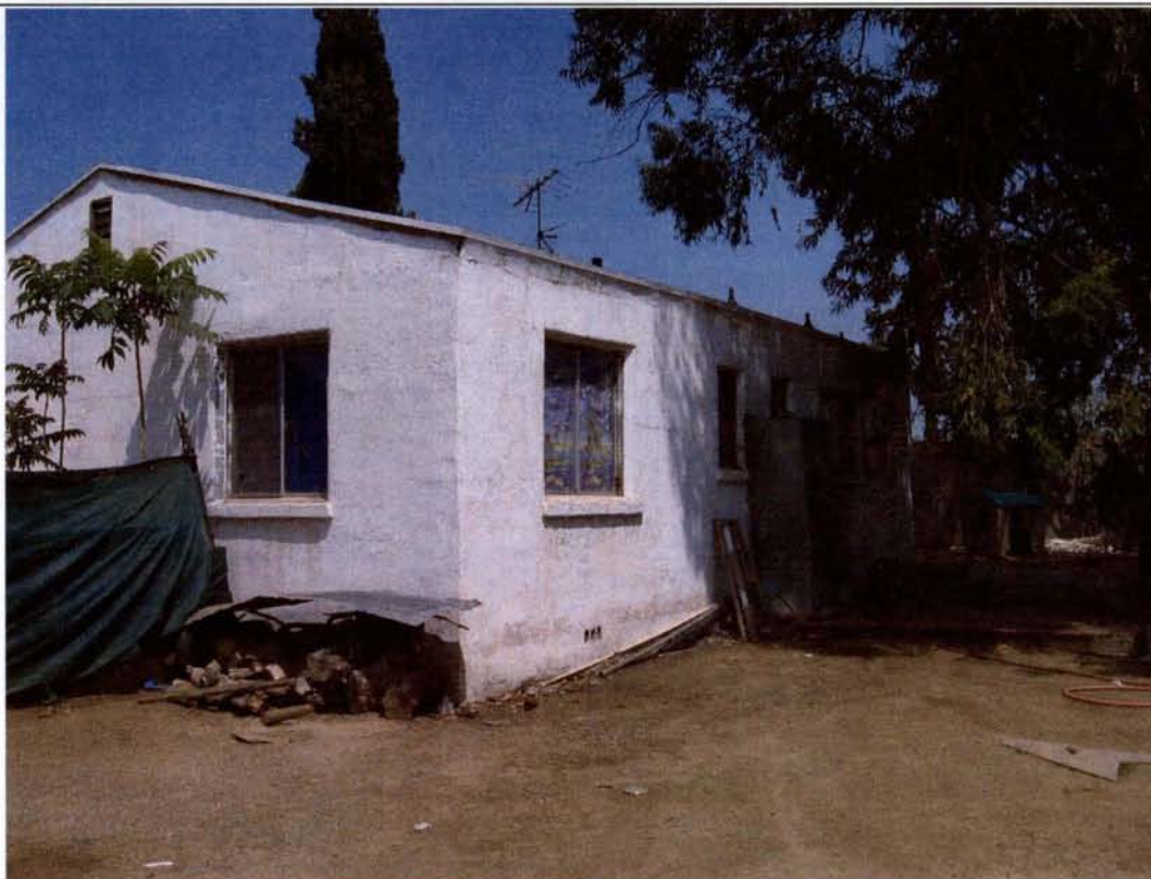
House A: Rear (east) elevation. View looking north.
