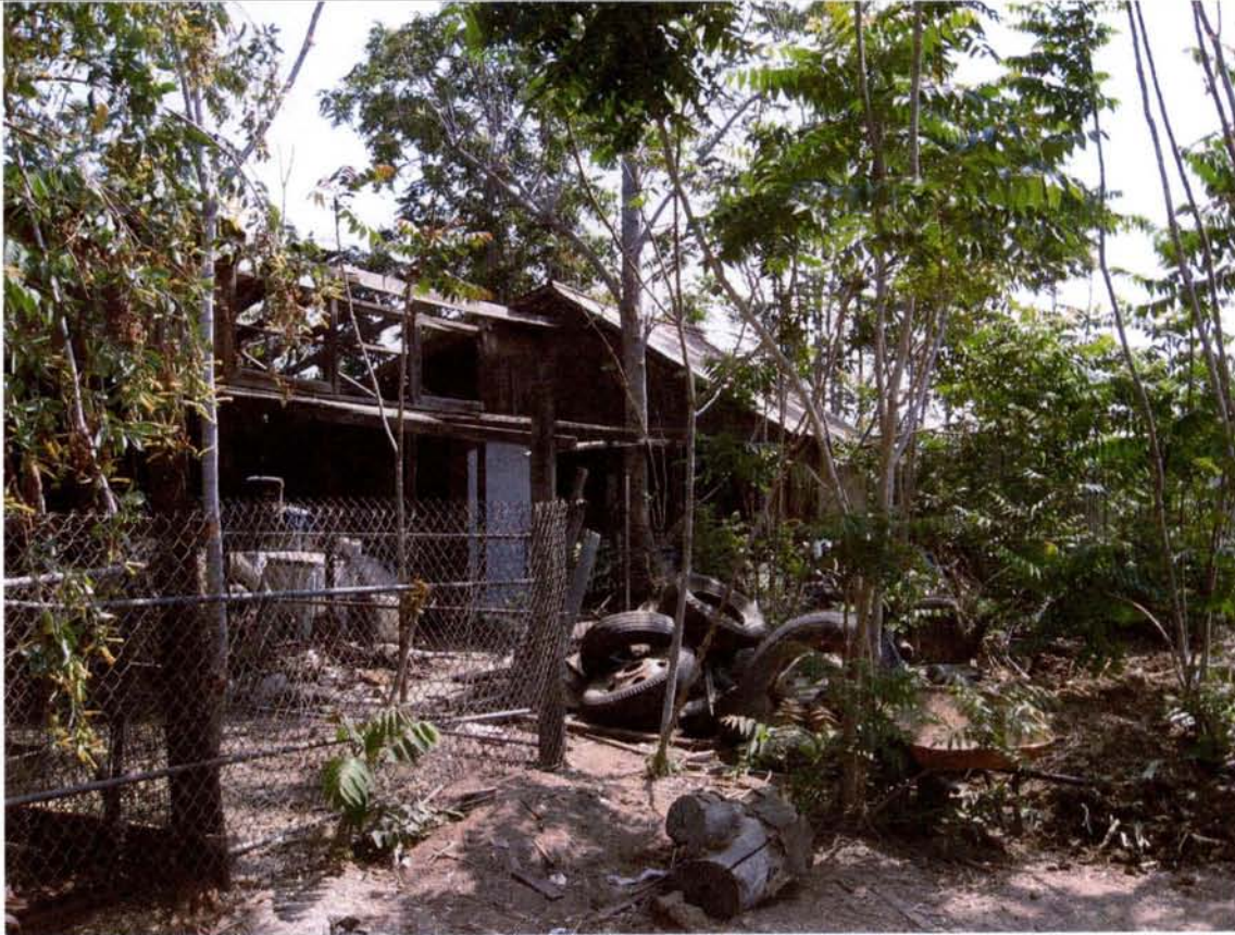
Gable barn: Front (west) elevation. View looking east.
