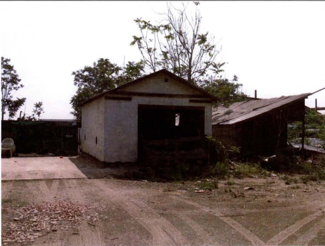
Garage: Front (west) elevation. View looking east.
