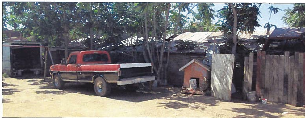
Poultry shed, north elevation, view to the southeast (5/17/15).
