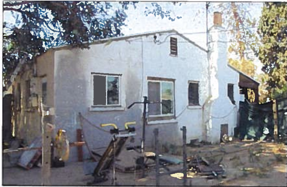
Primary residence, north elevation, view to the southwest (5/17/15).
