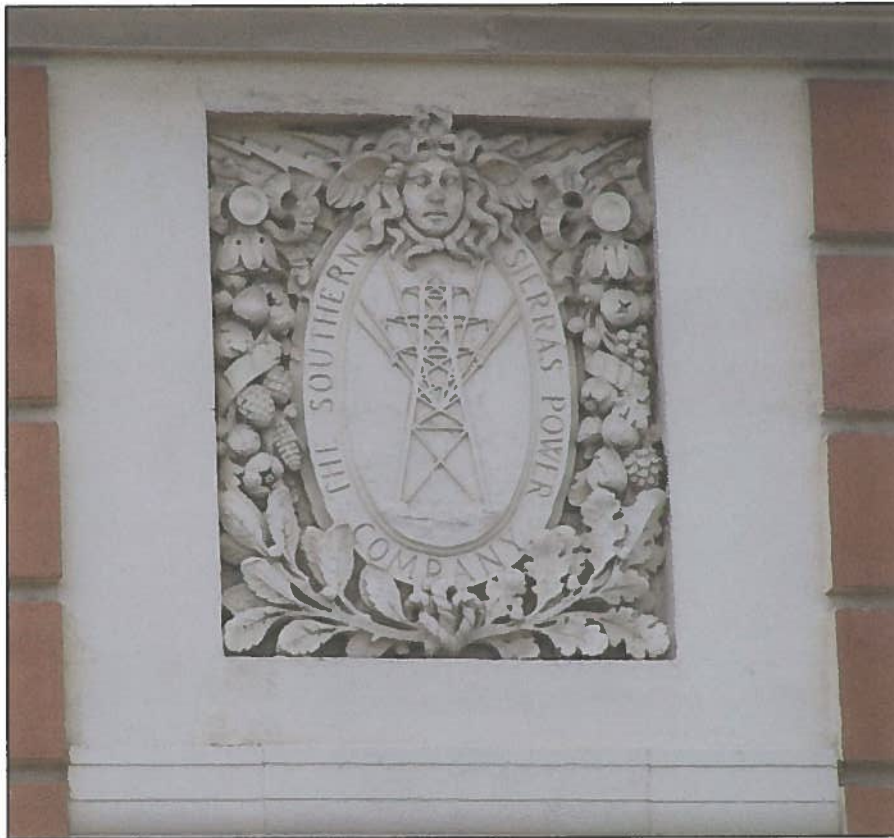
Photograph 5. Decorative embellishment in upper corners of First Steam Plant building to the right and the left of the main entrance. This building housed a 5000hp motor that generated electricity beginning in 1911. The building should be recorded as a separate property and should be considered significant at the State and Local levels.
