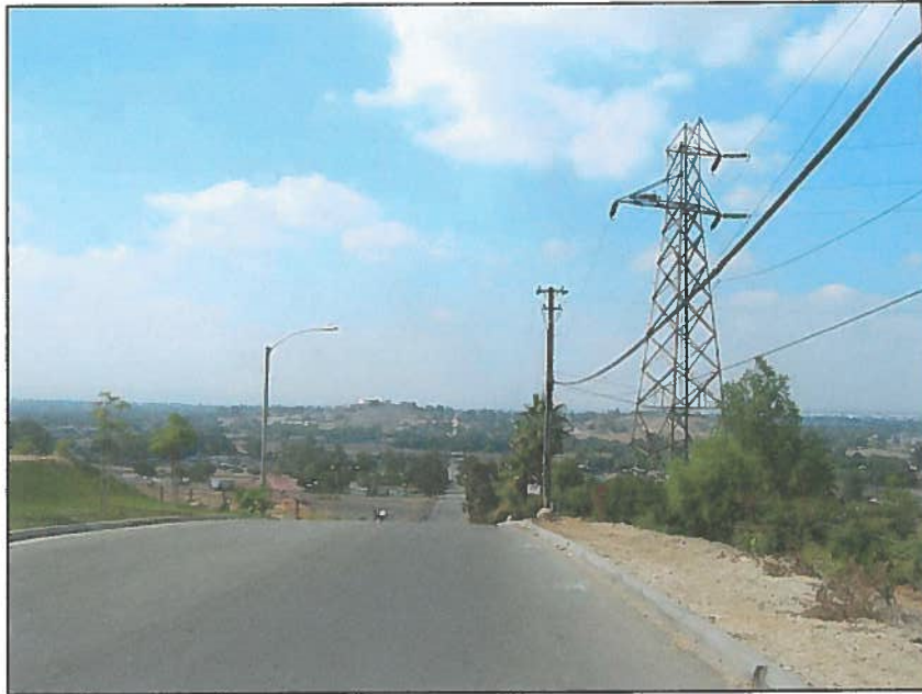
Photograph 2: View west of the tower and right-of-way east of the corner of 54 th and Agate Street, Riverside County. Pedley Road in the distance. Tower allows a bend in the lines. The lines at this point are probably not electrified.
