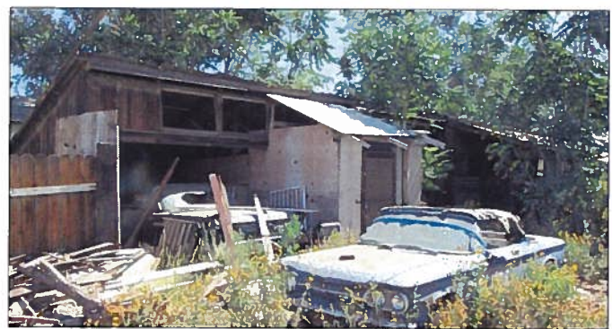
Poultry shed, south elevation, view to the northeast (5/17/15).
