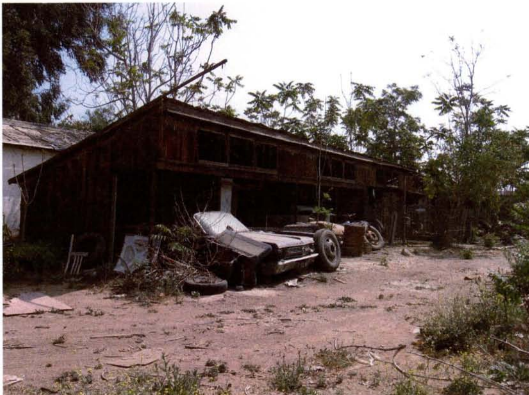
Poultry Shed: Front (south) elevation. View looking northeast.
