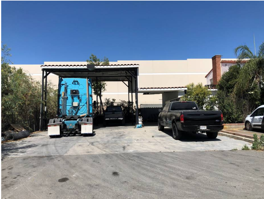
View of the covered parking area south of the Subject Property buildings.
