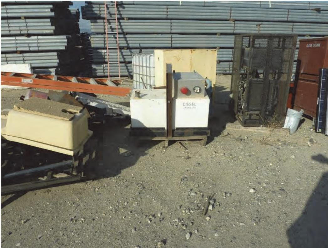
E-29. Looking north at portable, 60-gallon diesel AST with missing cap in Rig Runner area (11/19/2019).
