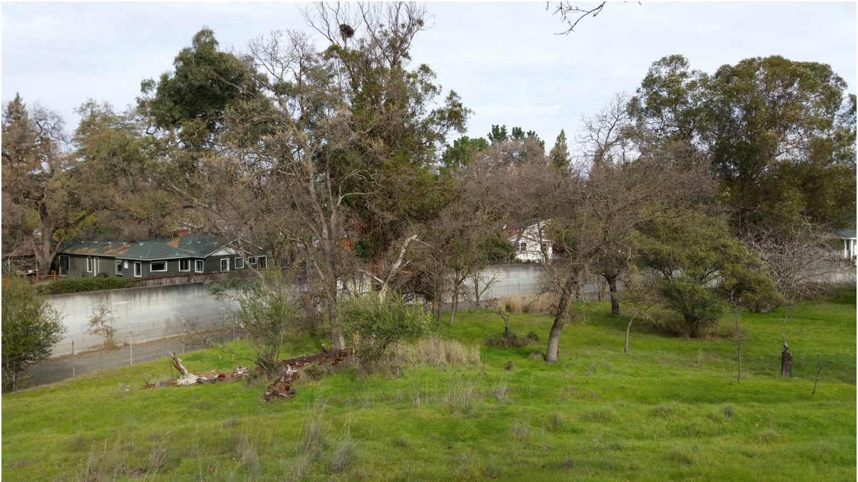
Photo 3. Looking west toward Walnut Creek (concrete-lined channel).
