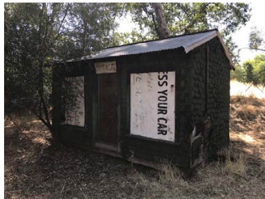
#18 NORTH ELEVATION OFFICE
