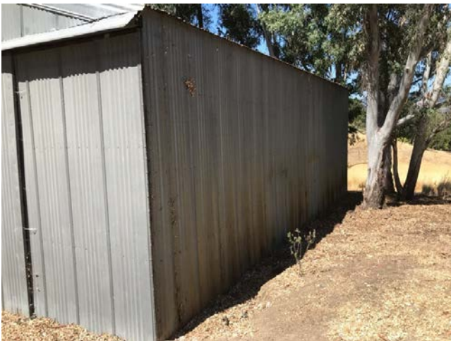
North elevation metal shed
