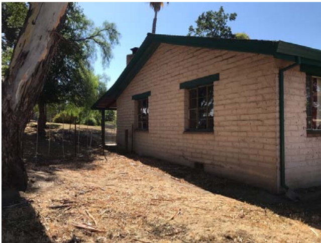
North elevation residence
