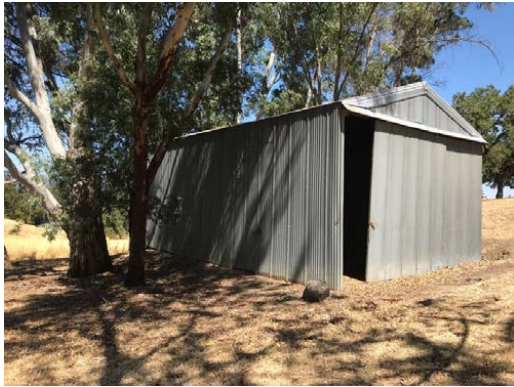
#15 SOUTH AND EAST ELEVATION METAL SHED
