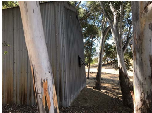
#16 NORTH ELEVATION METAL SHED
