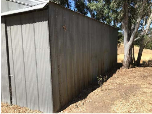
#13 NORTH ELEVATION METAL SHED
