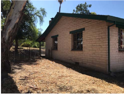
#1 NORTH ELEVATION RESIDENCE
