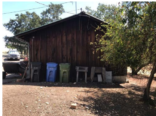
#12 WEST ELEVATION GARAGE/WELL HOUSE
