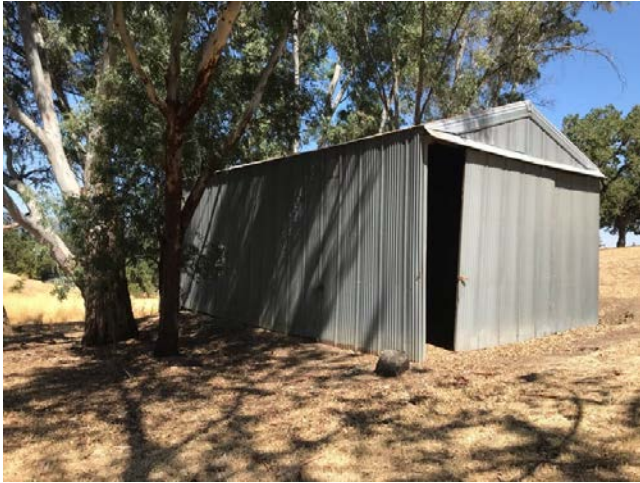
South and east elevation metal shed
