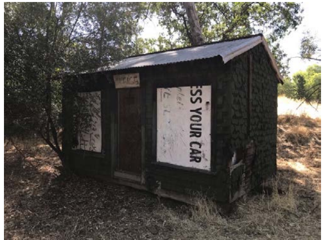
North elevation office
