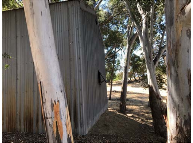
North elevation metal shed
