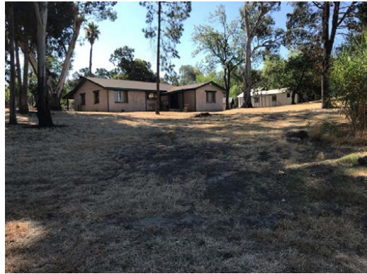
#34 SUSPECTED SEPTIC AREA
