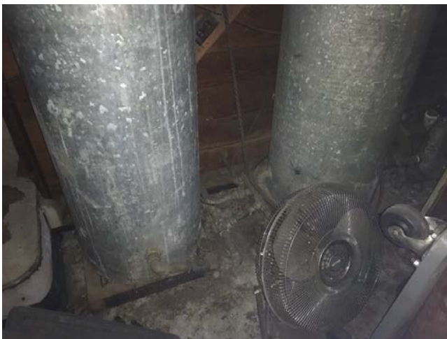
Well pressure tanks
