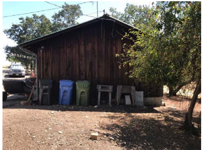
West elevation garage/well house
