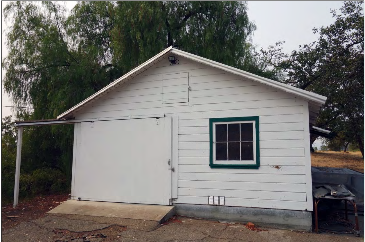
Figure 28: Southeast Façade, Building 2
