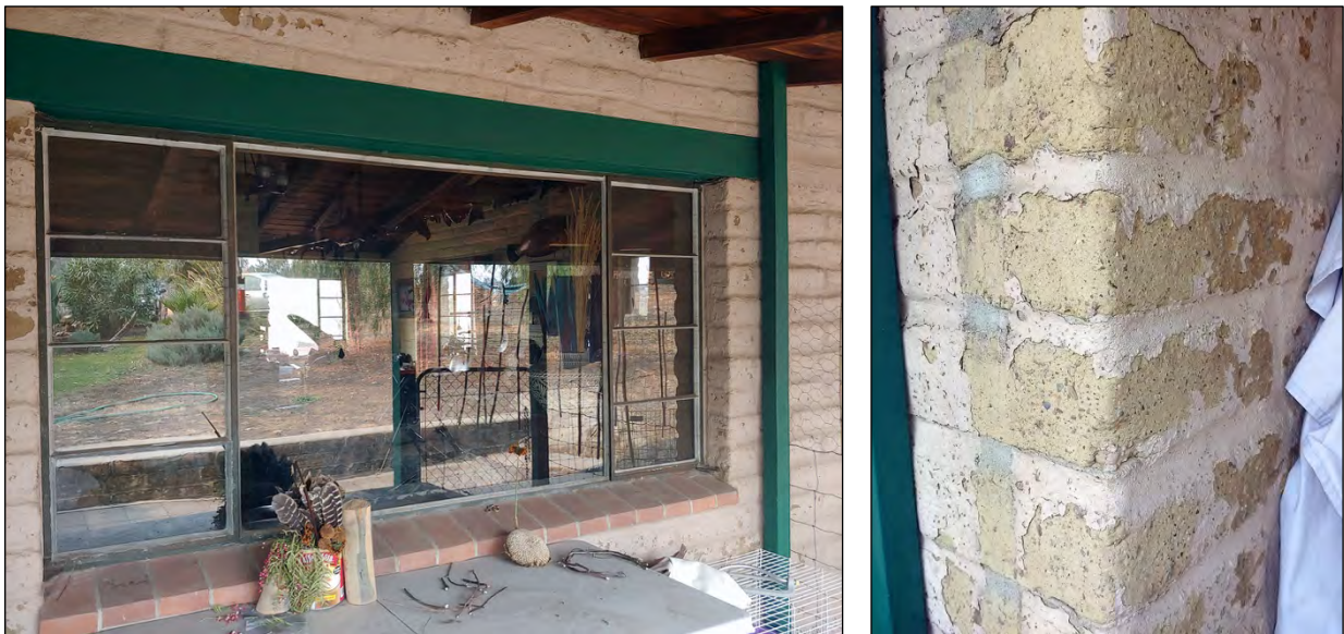
Figure 19: at left, window detail showing lintel; at right, adobe brick detail
