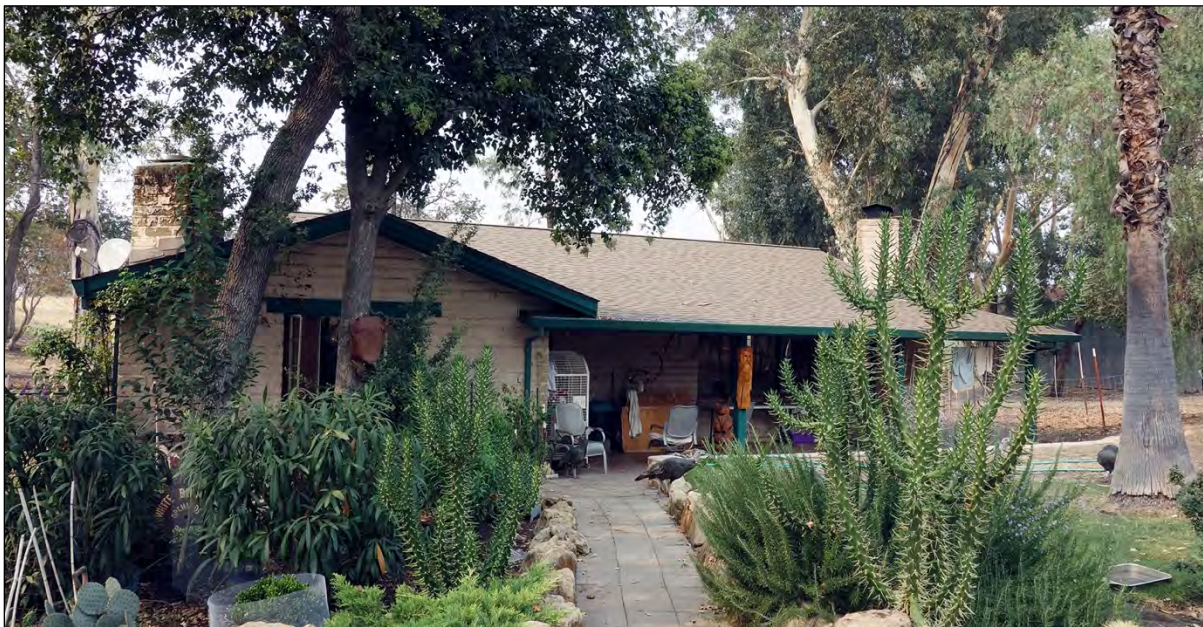
Figure 13: East Façade, Main House
