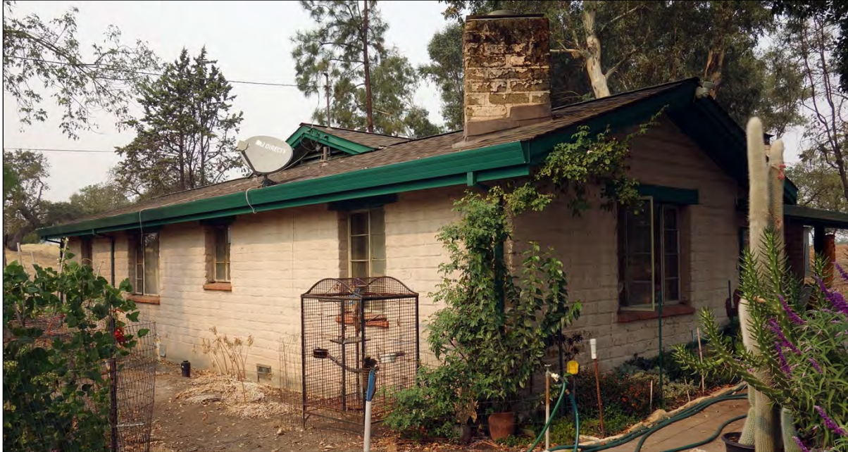
Figure 16: Southeast corner of main house showing South façade
