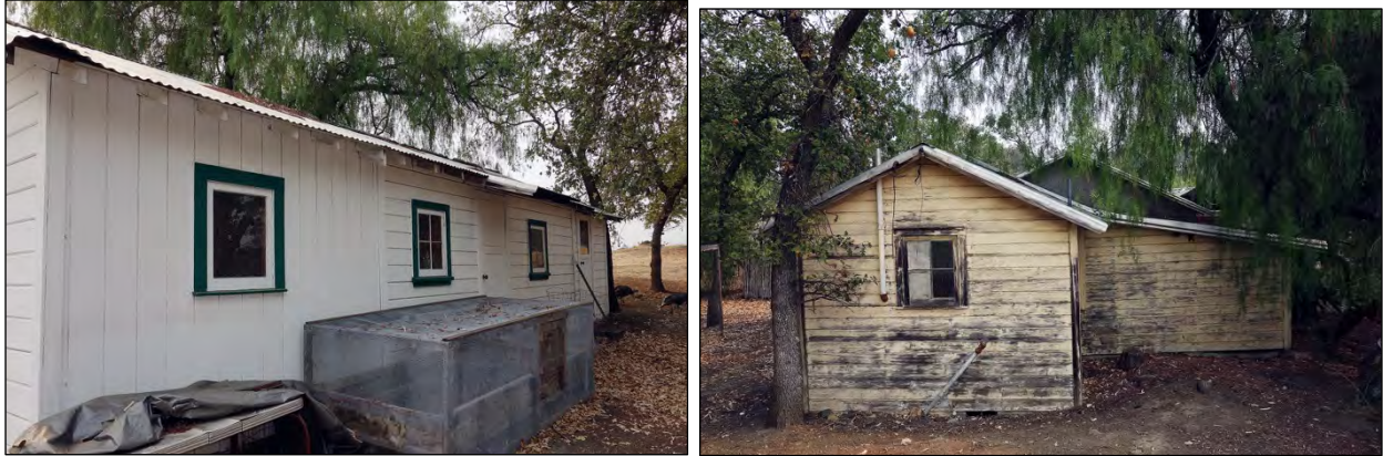
Figure 27: at left, Northeast Façade, Building 2 ; at right, Northwest Façade, Building 2
