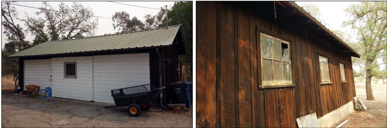
Figure 26: at left, North Façade, Building 1 ; at right, South Façade, Building 1
