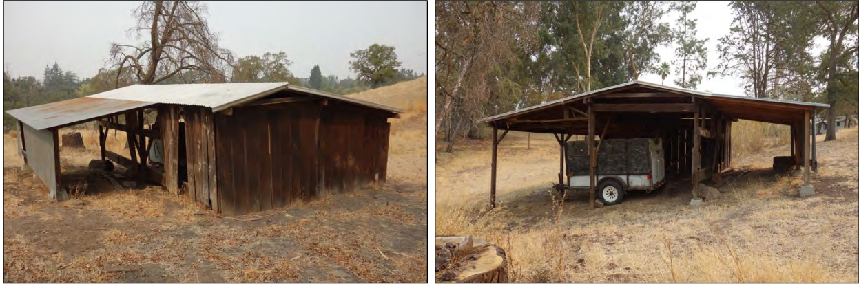
Figure 29: at left, Southeast corner, Building 4 ; at right, West side, Building 4
