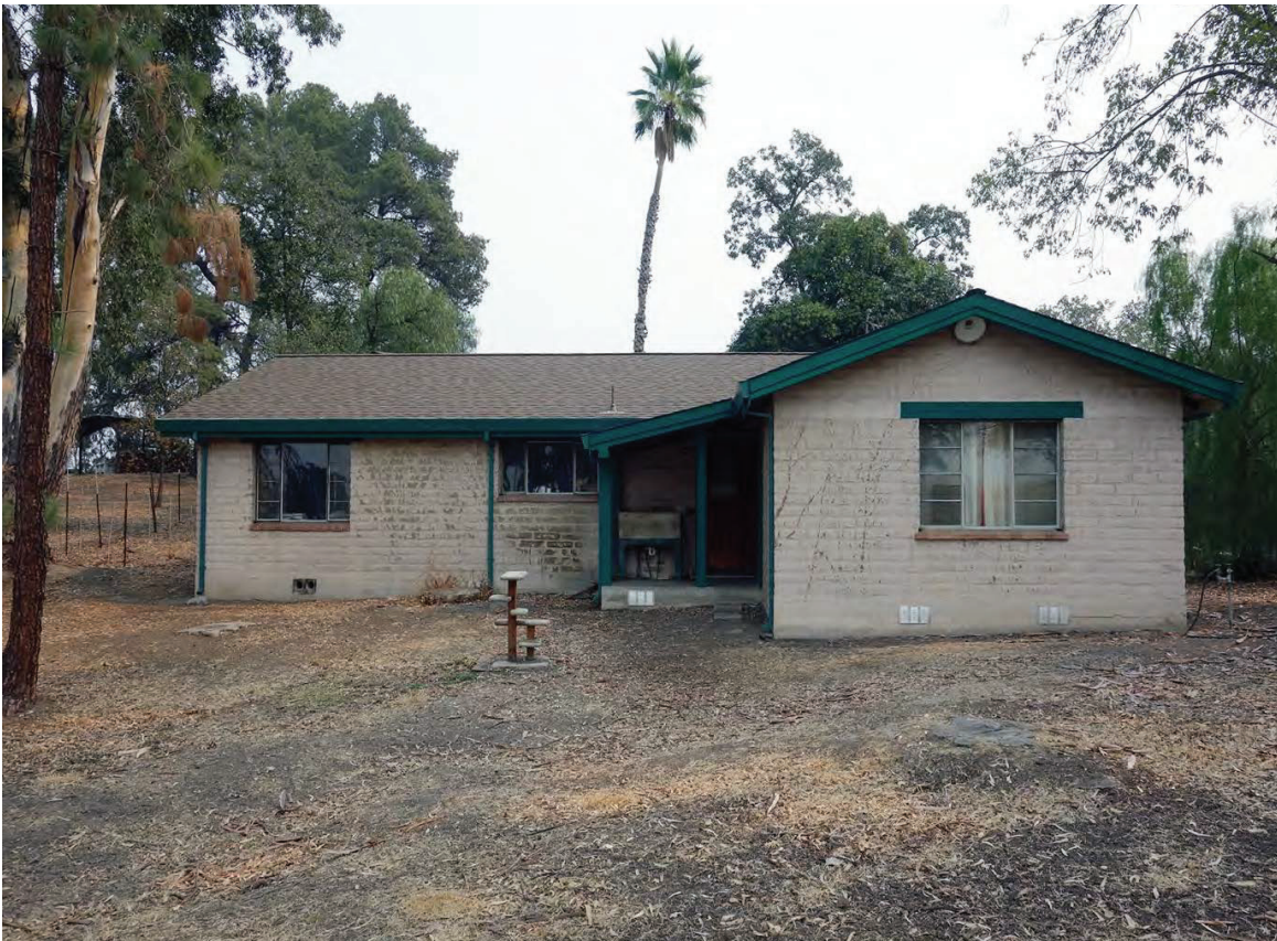
Photo 8: Rear of Single-Family Home/West Facade
