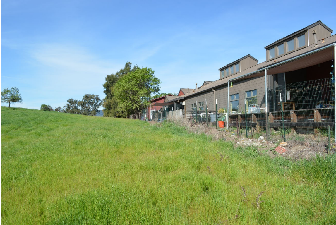
Location 26: Looking West along Seven Hills School Boundary
