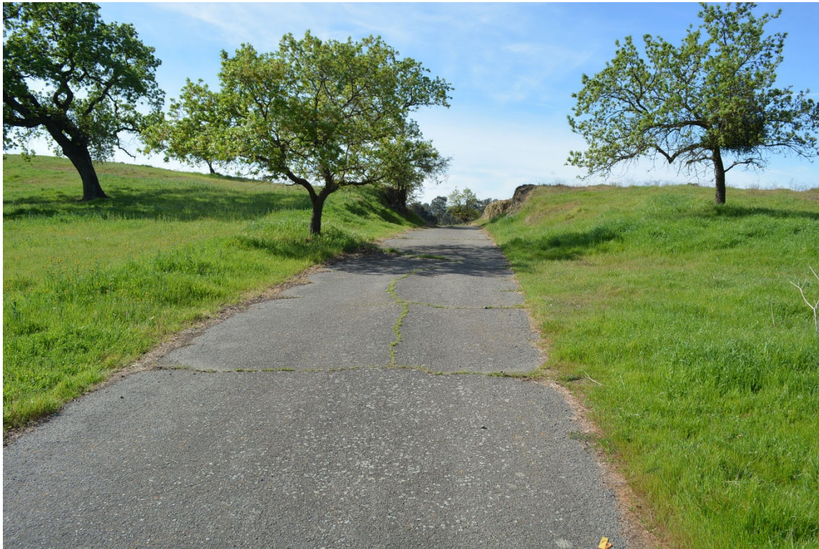
Location 28: Looking South from Seven Hills School Along Ranch Road
