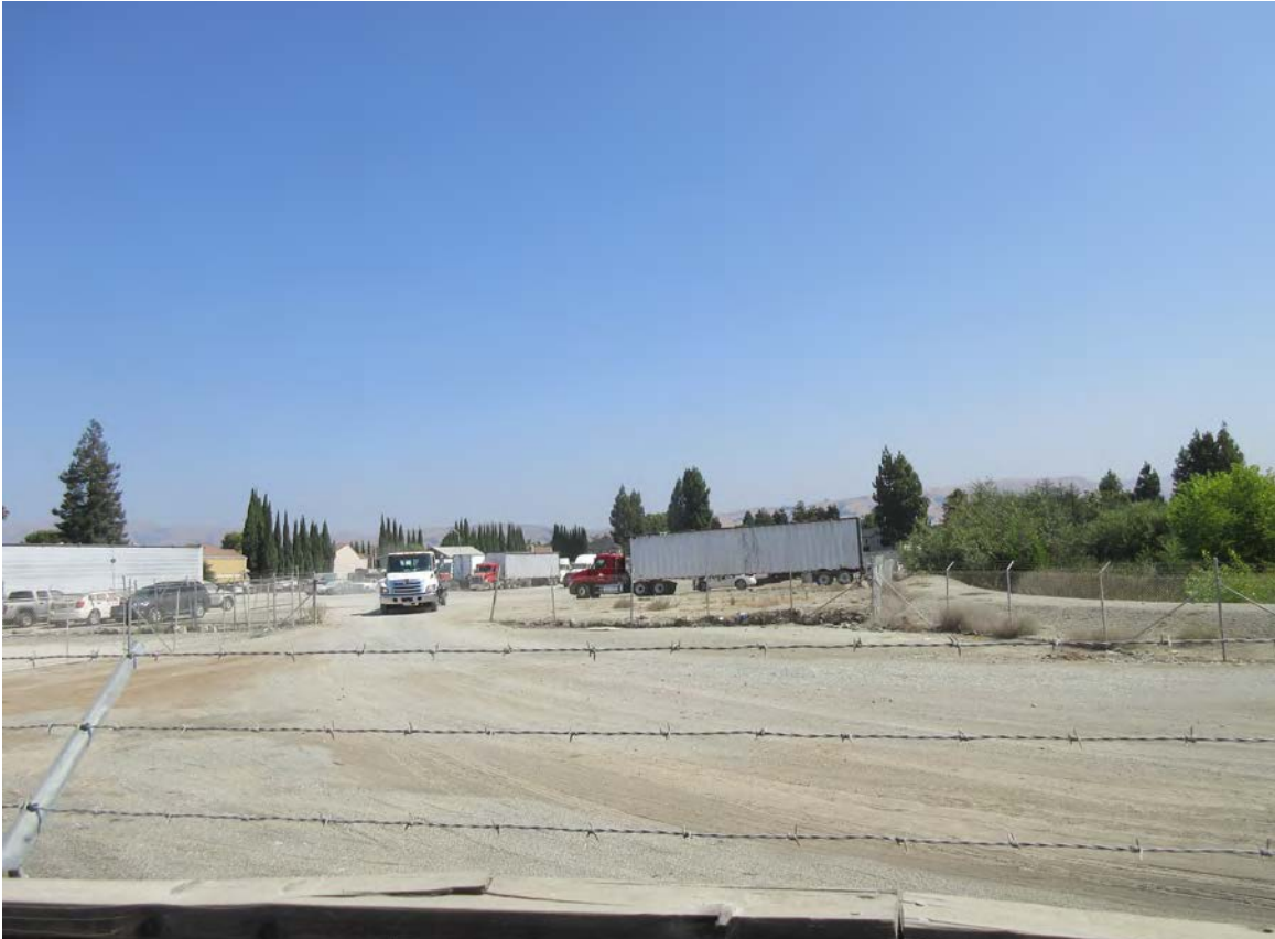
Photo 1: View of existing project site, facing south.
