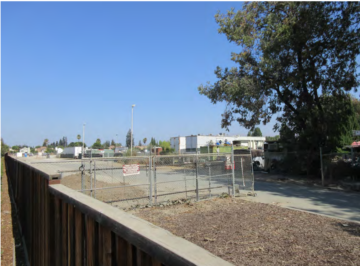
Photo 2: View of existing project site, facing east.
