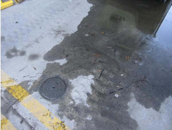
Photograph 7. Concrete-filled oil-water separator at AT&T (below standing rain water).
